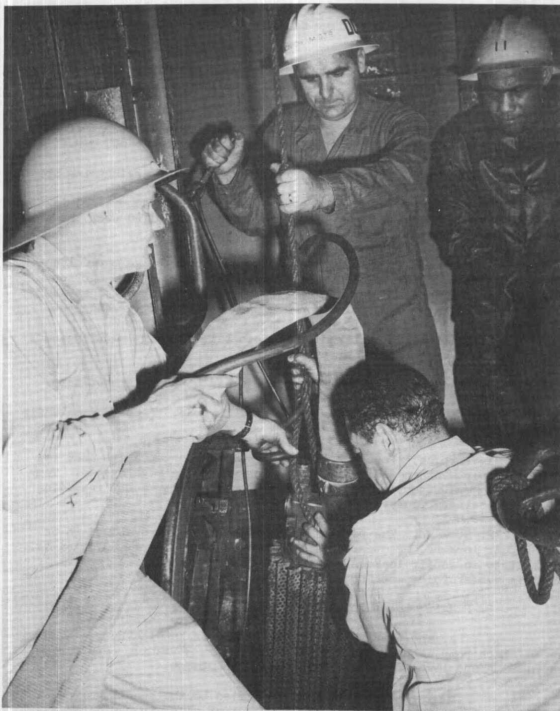
LOWERING PORTABLE ELECTRIC SUBMERSIBLE PUMP, WITH BASKET STRAINER.
