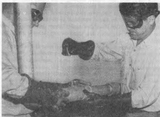
RETAINING COVER goes over the glass fiber mat. Ordinary brown wrapping paper provides sufficient outer protection. Plastic patches can be used on shipboard pipelines with pressures up to 300 p. s. i.
