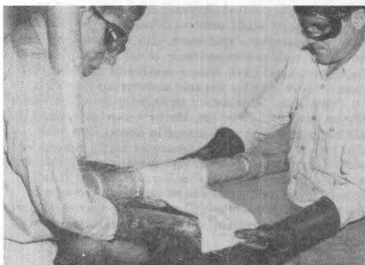
GLASS FIBER MAT is placed over the plastic tape. The mat is saturated with chemically heated plastic resin compound. As the resin cools, the various layers harden into a firm, watertight patch.
