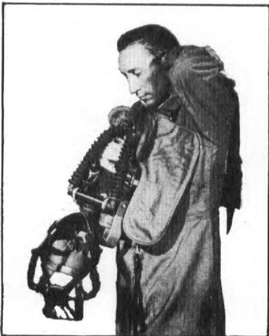
hand holding apparatus, with other hand grasp D-Ring assembly with breathing tubes hanging forward. Put breast plate on chest and head through v-shaped opening formed by the crossing of two straps attached to breast plate.
