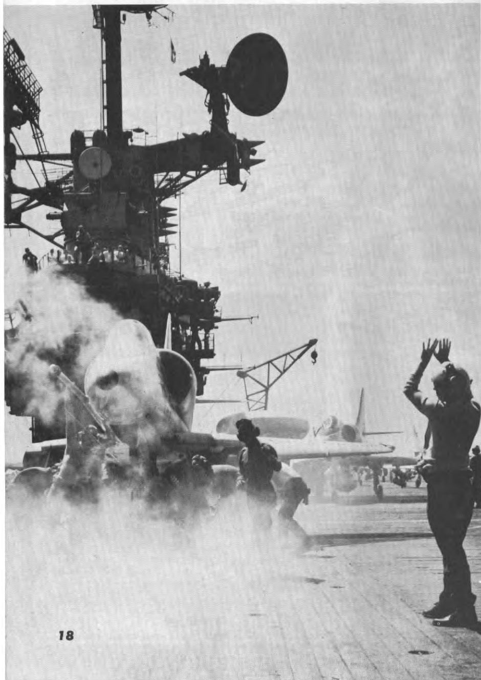
← SLOT MACHINE —Cat men, USS Hancock (CVA 19), attach bridle to Skyhawk as the steam pressure is built up.
