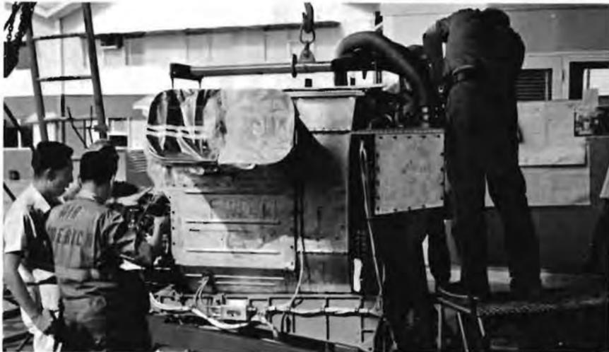
2. Left side of a Twin-Pac powerplant for an S-58T being assembled at Udorn. Large duct at the top is twin exhaust outlet.
