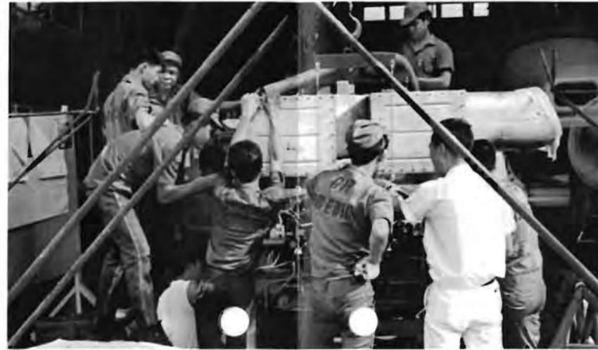
4. Air America mechanic personnel working on a Twin-Pac powerplant prior to installing it in an S-58T.
