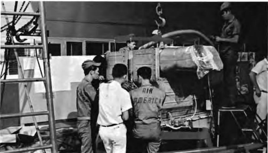
3. Air America leadman and mechanics prepare a Twin-Pac powerplant for installation in an S-58T.
