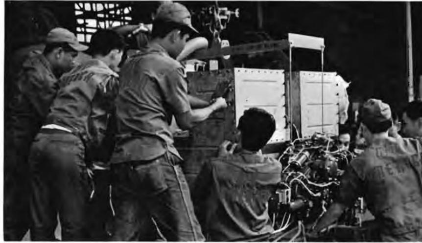
1. Air America mechanics assemble a Twin-Pac powerplant prior to installation in an S-58T.
