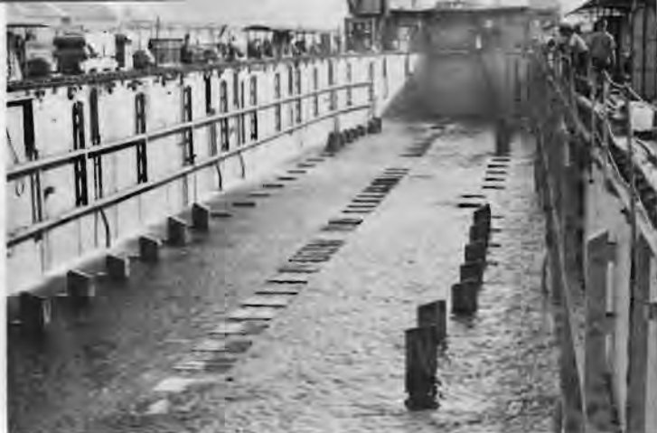
USS WINDSOR at work in Subic. Rt: Docking basin is lined with keel blocks which will support incoming ship.
