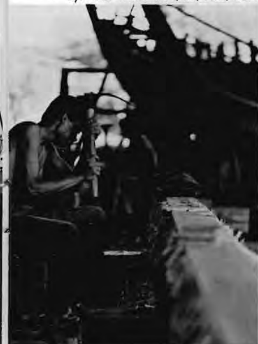
Young carpenter narrows a Sao log which will later be intricately carved before being used as beam in junk.
