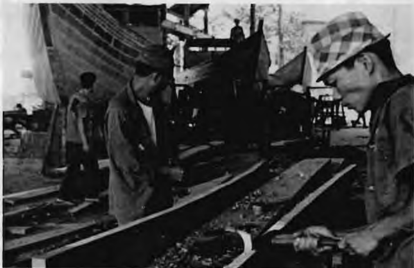
Hatchets and planes are used to complete one junk every seven weeks.
