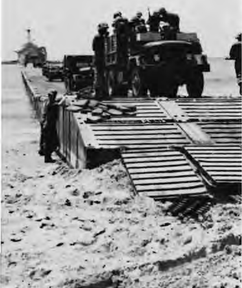
INSTANT CAUSEWAY — Support equipment is unloaded from Jerome County (LST 848) onto floating roadway.—Photo, R. Benjamin, JO1.
