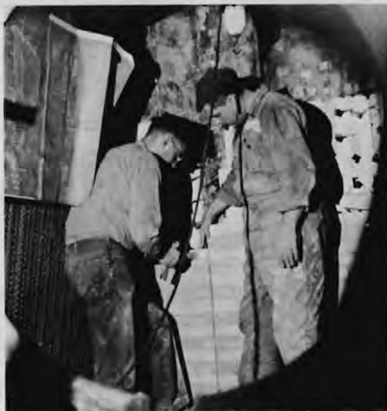
Firebrick is laid at expansion joint.
