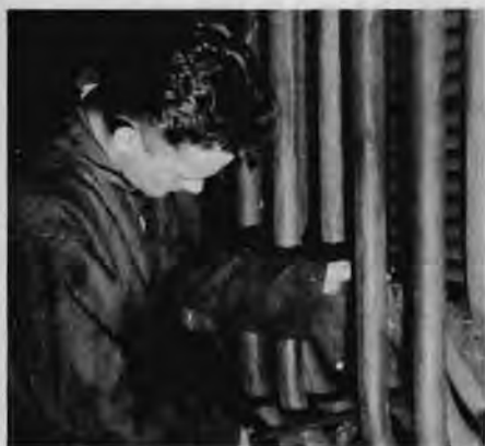
Superheater screen tubes are worked on.
