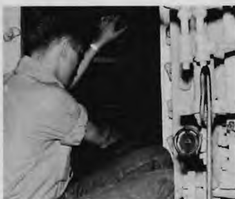
Cleaning diffuser on air register inside boiler.
