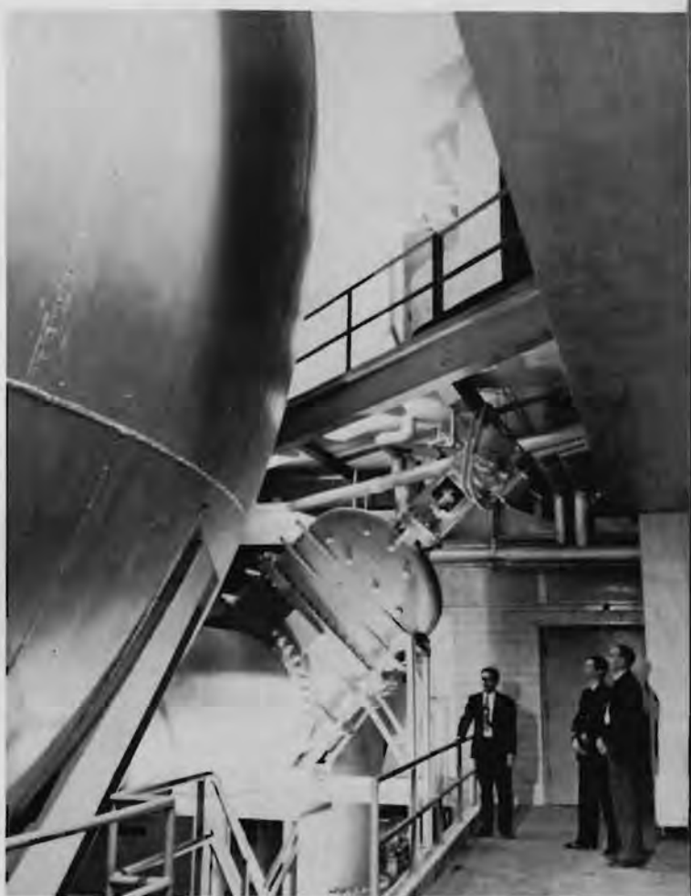
Steel vacuum sphere, dedicated in 1949, set former speed record for wind tunnel research. Below: Explosive developed by NOL allowed lunar module to descend to and ascend from the moon, thereby aiding in the success of Apollo 11.
