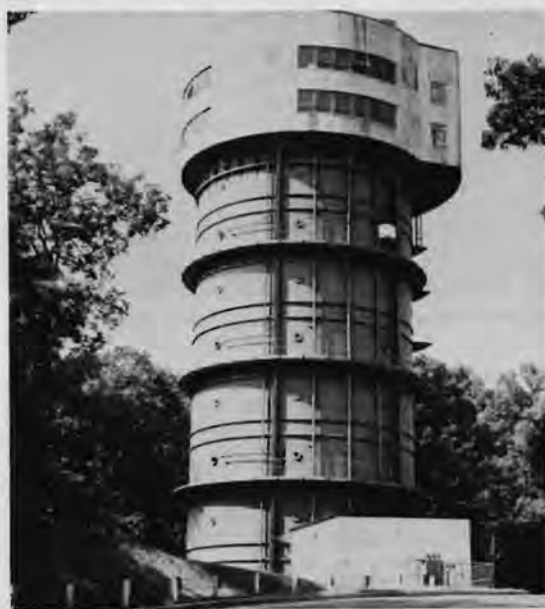
The 100-foot underwater weapons test tank at NOL holds some 1½ million gallons of water.
