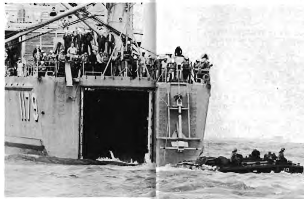
UPHILL CLIMB —Truck tests traction of bow ramp of new LST. Below: Tank landing ship USS Newport (LST 1179) lies at anchor off coast of Virginia. Rt: Landing craft emerges from stern during evaluation tests on underway launching.
