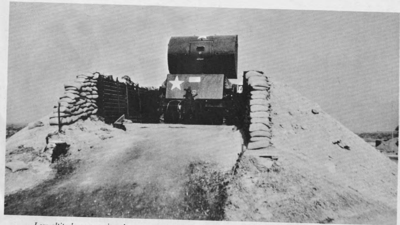
*Low altitude enemy aircraft are tracked with the Continuous Wave Acquisition Radar (CWAR)*
