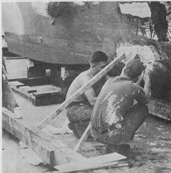
PATCH UP —DC2 John A. Dankson and DC3 Ray Beets of the APL-55's Damage Control Division fiberglass a Mark II PBR hull.
