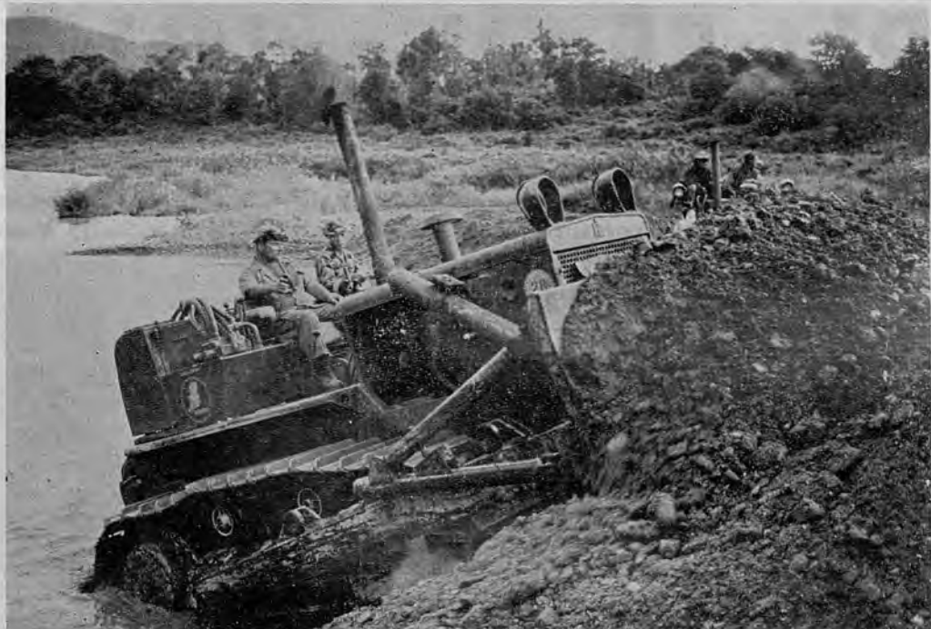
TONS OF GRAVEL —Equipment Operator First Class Leon L. Snider uses a bulldozer to scrape gravel taken from the Pon River into piles which will then be picked up by front end loaders and put into trucks. (Official U.S. Navy Photo)
