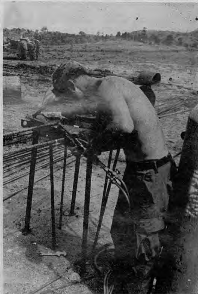
TWO JOBS —Hospital Corpsman Second Class Thomas J. King cuts reinforcing bars used in constructing concrete machine gun bunkers at Lang Vei. Each Seabee had to perform the duties of at least one other man in addition to his own. (Official U.S. Navy Photo)
