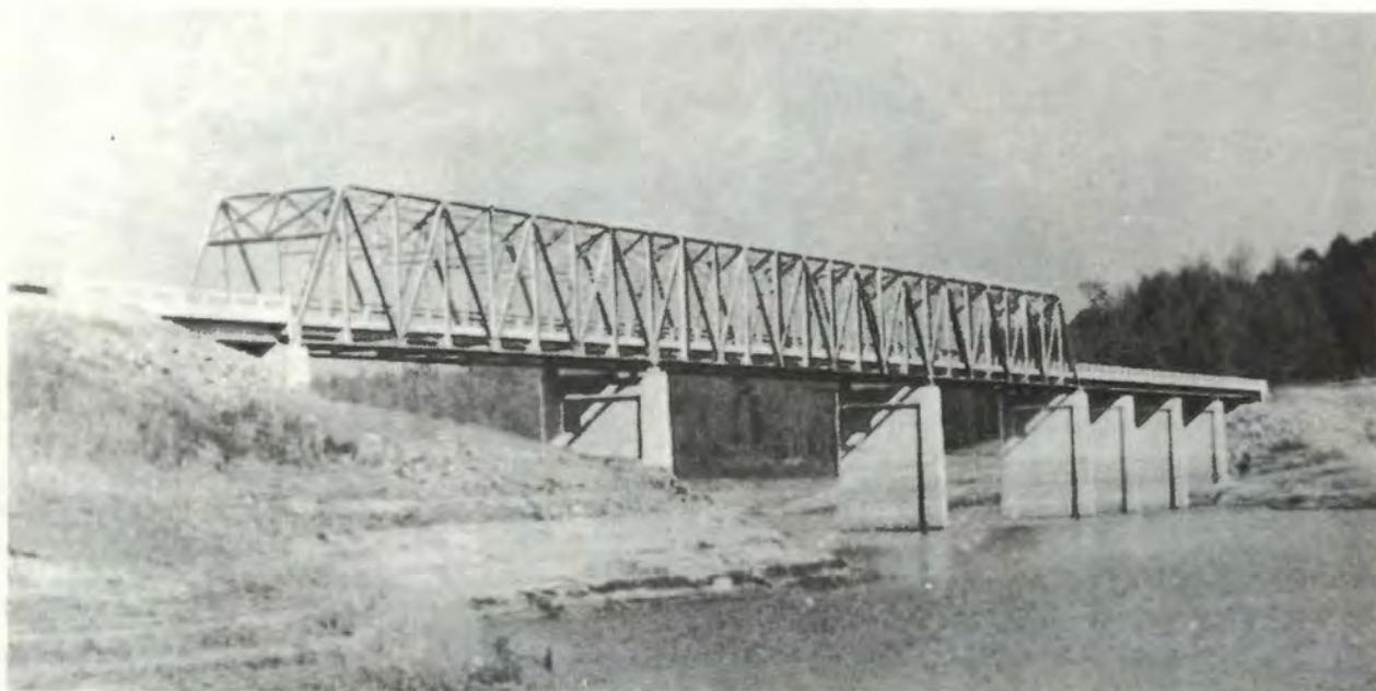
Figure 3-36. Typical steel through truss bridge (Warren type).
