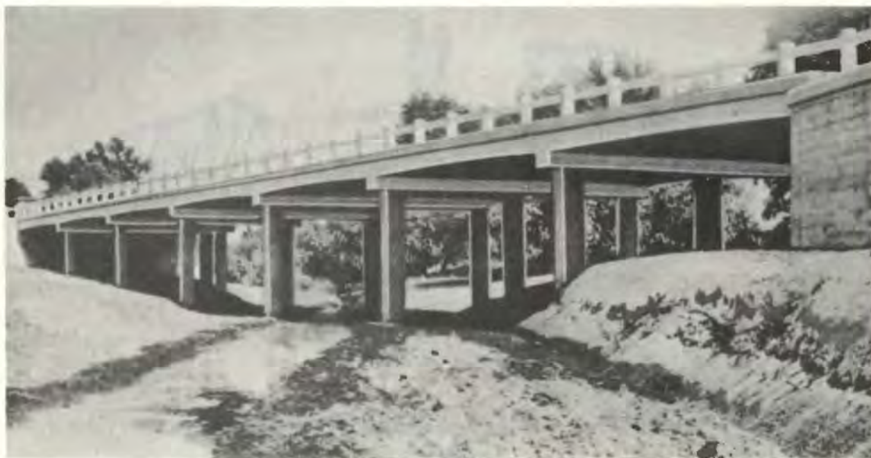
Figure 3-22. Typical concrete slab bridge.
