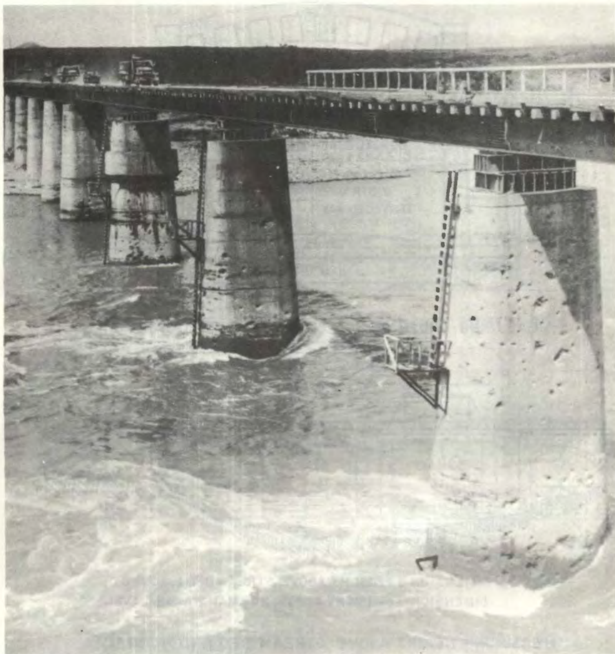
Figure 3-18. Typical solid concrete pier.
