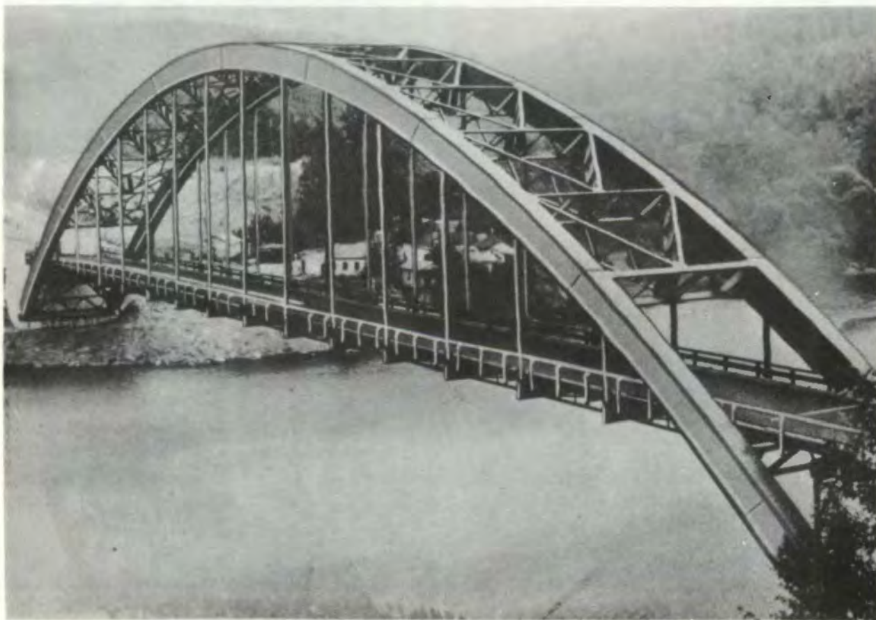
Figure 3-50. Steel arch bridge, through type.
