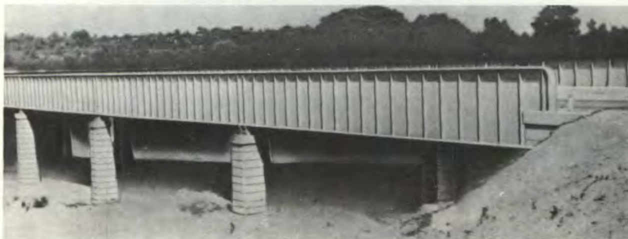
Figure 3-41. Through type girder bridge.
