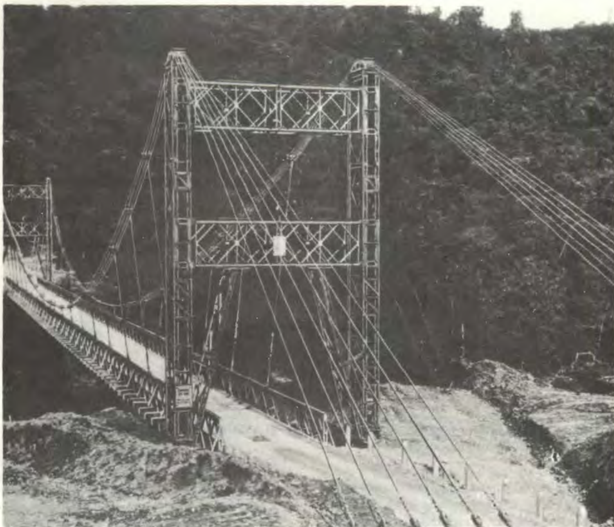
Figure 3-54. Steel suspension bridge.
