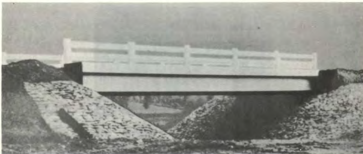
Figure 3-27. Simple stringer bridge with steel I-beam stringers and concrete slab flooring.
