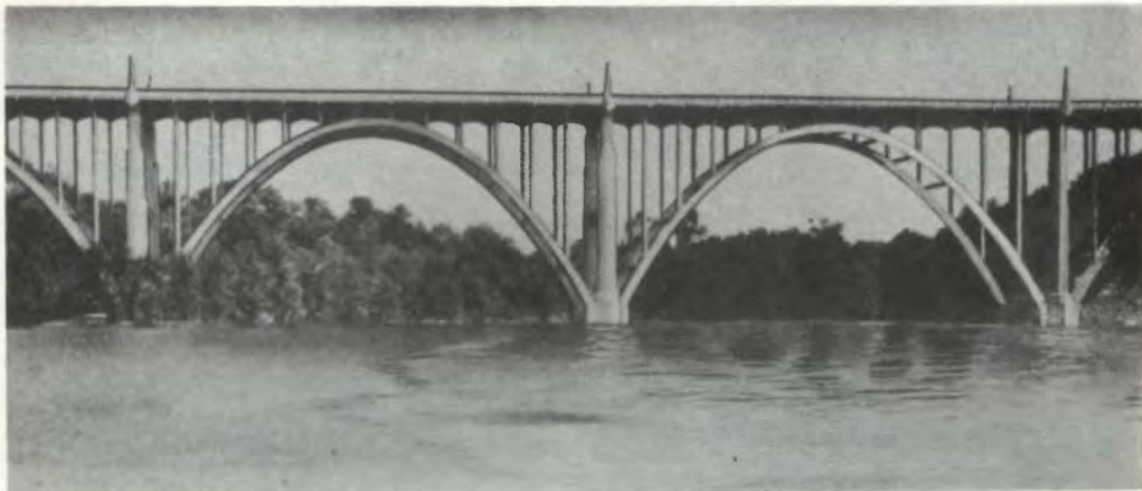
Figure 3-49. Steel trussed arch bridge, deck type.
