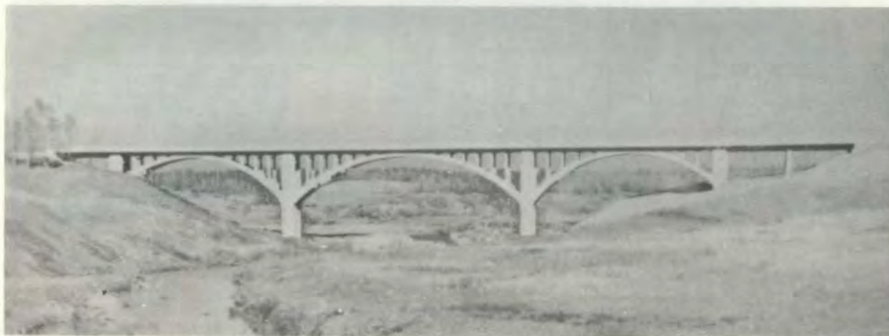
Figure 3-47. Typical open spandrel concrete arch bridge.
