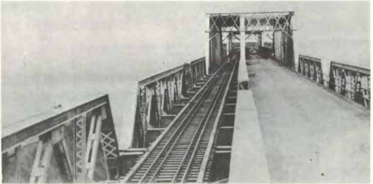
Figure 3-38. Pony truss and through truss forming combination bridge.
