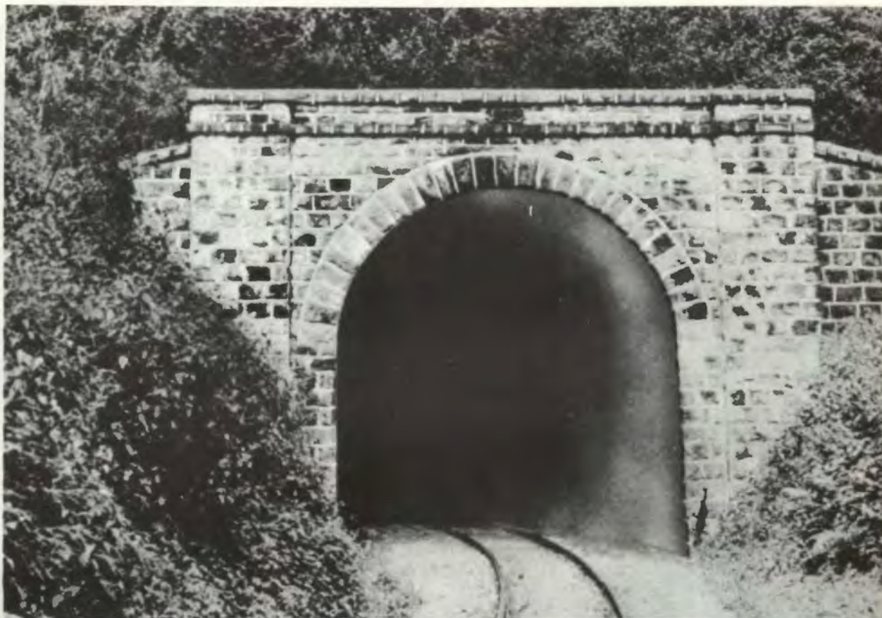
Figure 2-21. Typical masonry portal.
