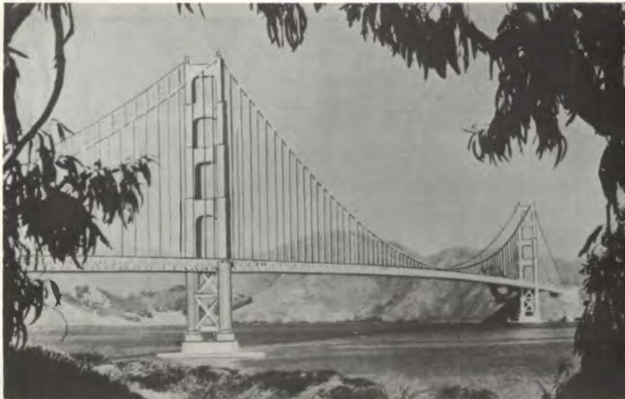
Figure 3-52. Suspension bridge with steel cable, steel reinforcing truss, steel floor beams, and external sway bracing.
