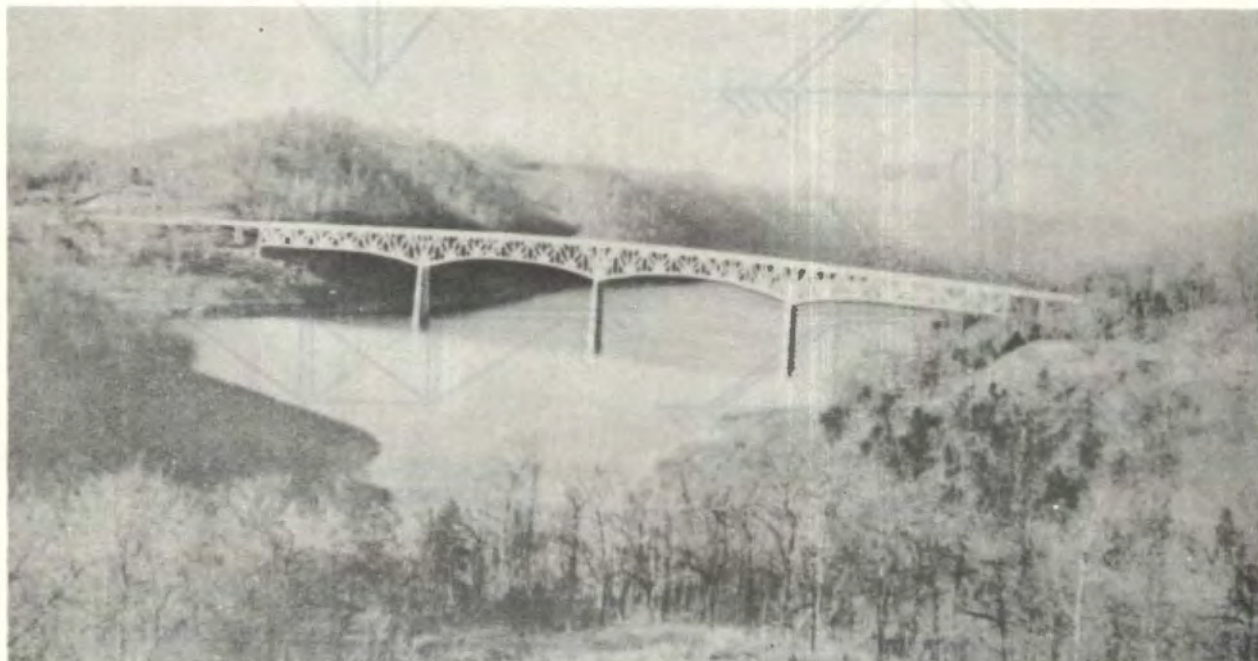
Figure 3-34. Typical steel deck truss bridge.
