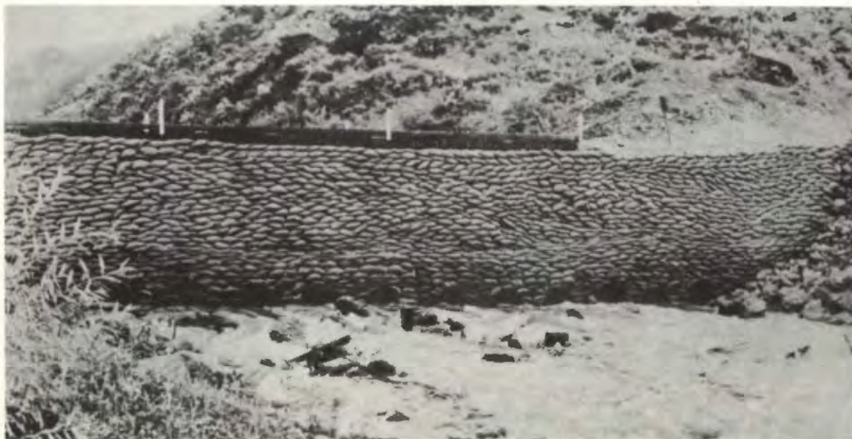
Figure 2-65. Causeway with culverts.
