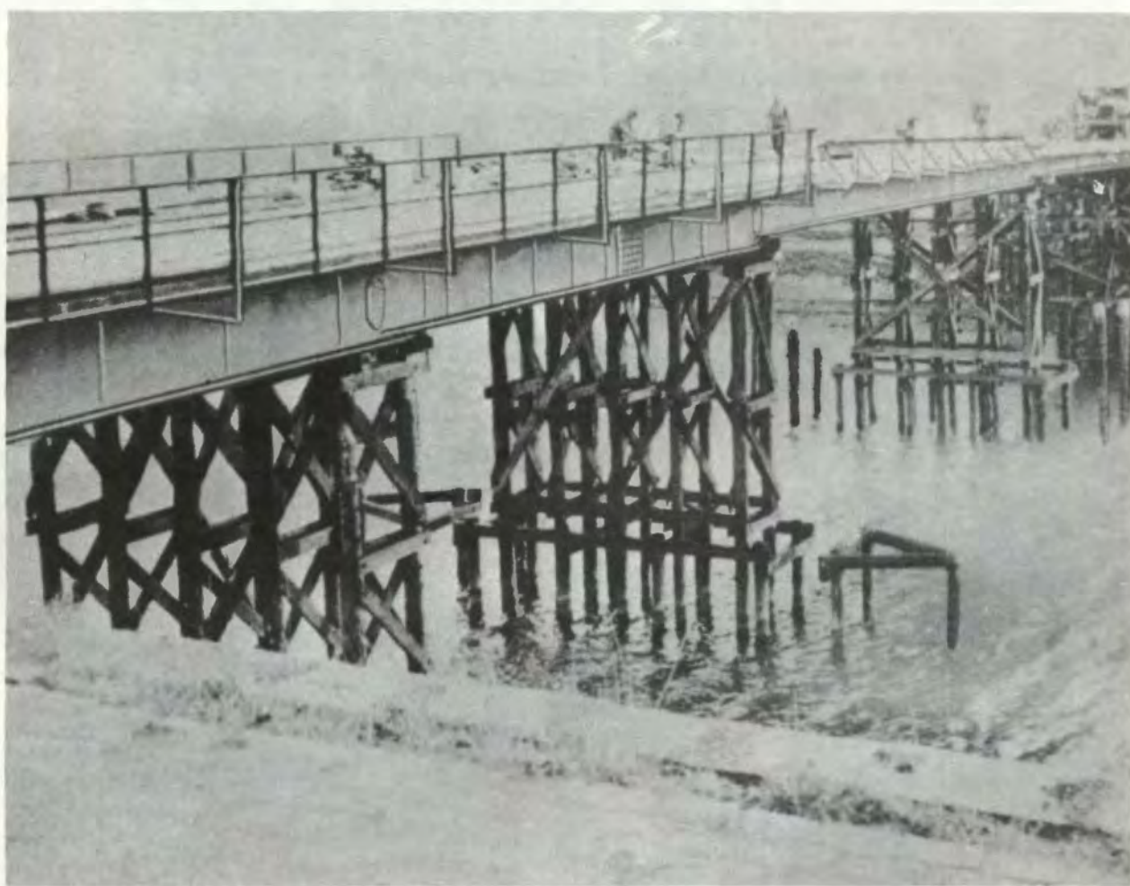
Figure 3-26. Simple stringer bridge with steel I-beam stringers and timber flooring.
