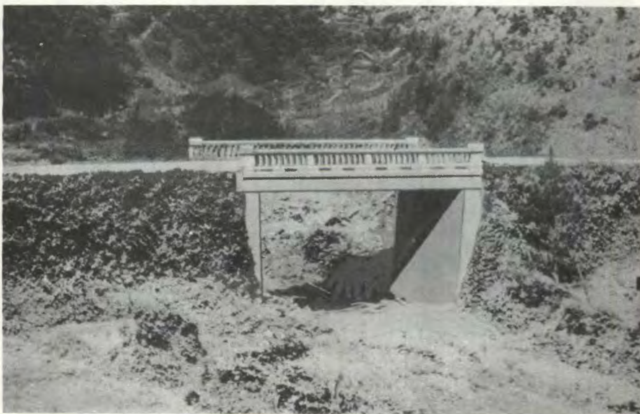
Figure 3-28. Typical single span concrete bridge.
