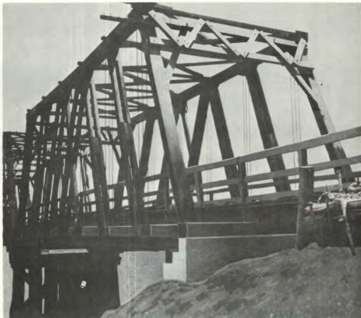
Figure 3-35. Typical timber truss bridge.
