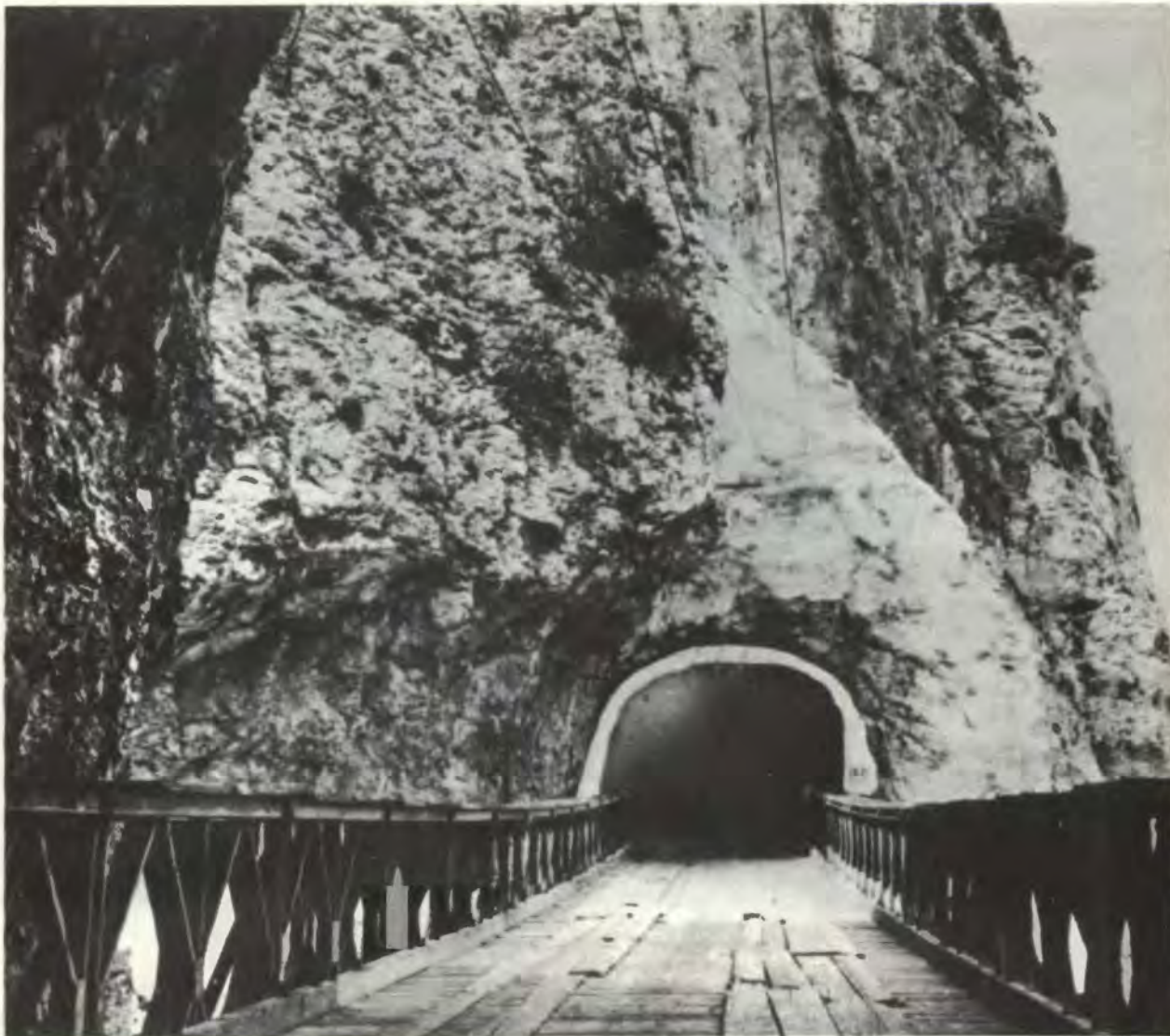
Figure 2-20. Typical concrete-lined tunnel.
