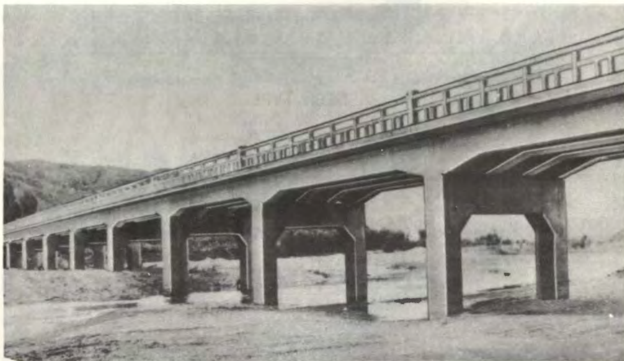
Figure 3-30. Typical multispan concrete T-beam bridge.
