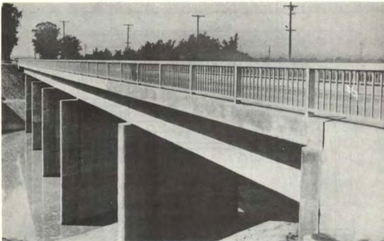
Figure 3-29. Typical concrete bridge.
