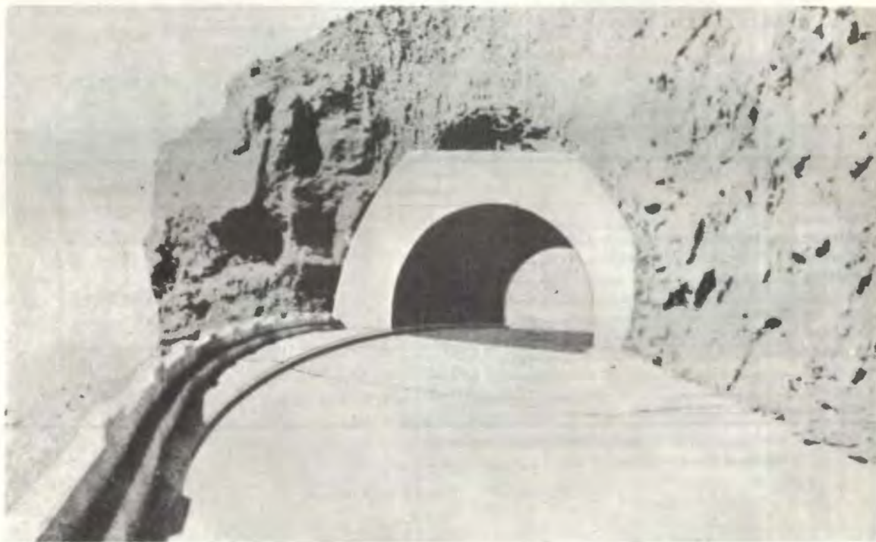
Figure 2-24. Tunnel with curved horizontal alinement.
