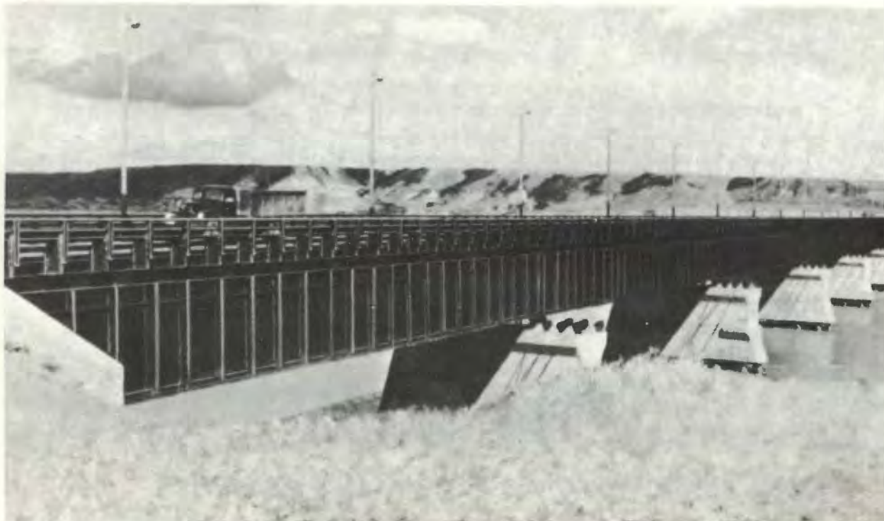
Figure 3-40. Typical multispan deck type plate girder bridge.
