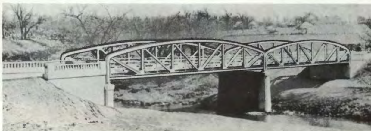
Figure 3-37. Pony truss highway bridge.
