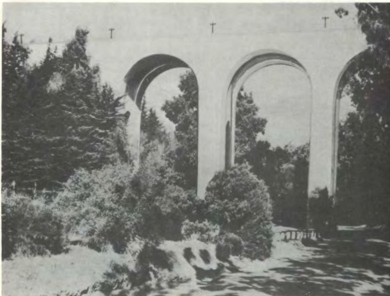
Figure 3-46. Typical solid concrete arch bridge.
