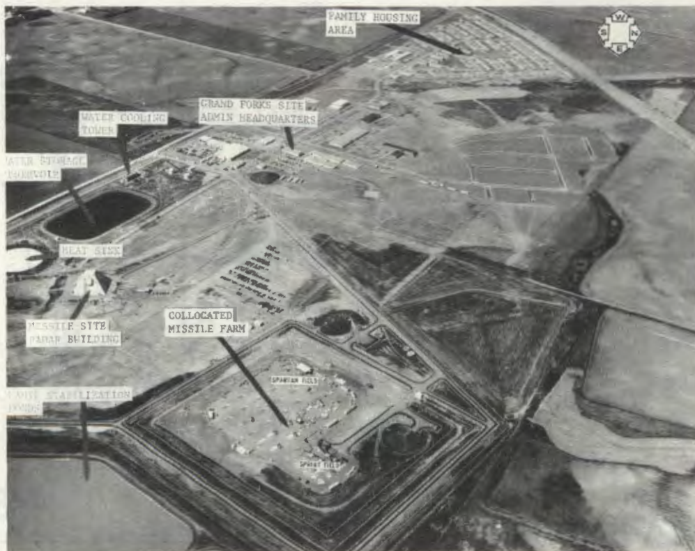
Figure 8. Missile direction center complex.
