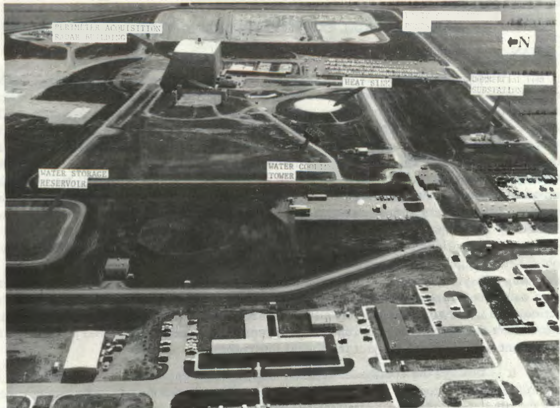
Figure 10. Perimeter acquisition radar site assembly complex.
