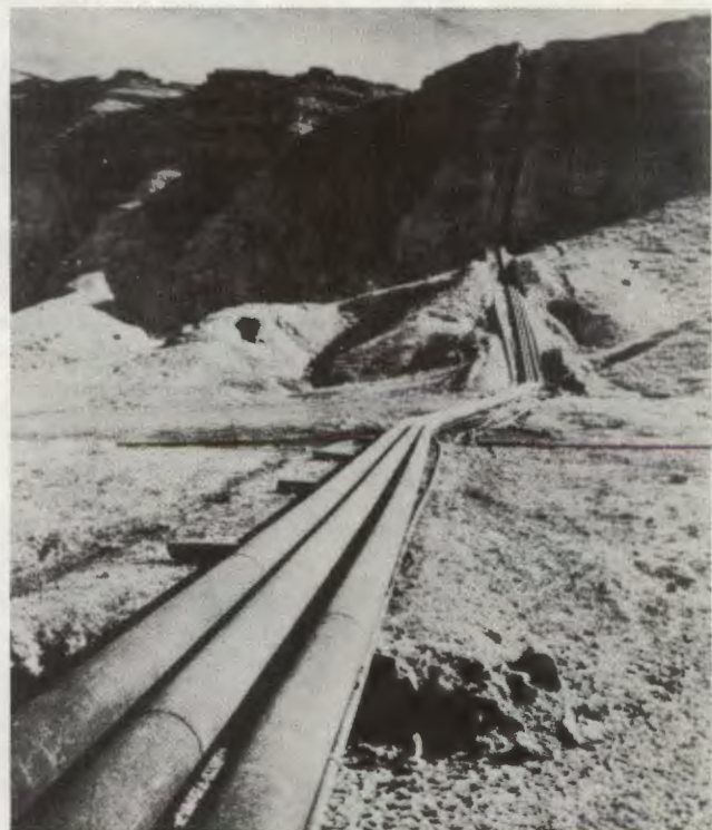
Figure 5-20. Pipeline laid above ground.
