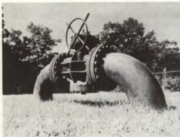
Figure 5-22. Cutoff valve.
