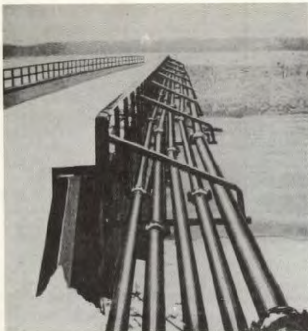
Figure 5-21. Pipeline crossing stream on existing bridge.
