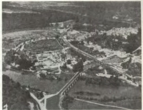
Figure 5-32. Aqueduct carrying a waterway over a river.
