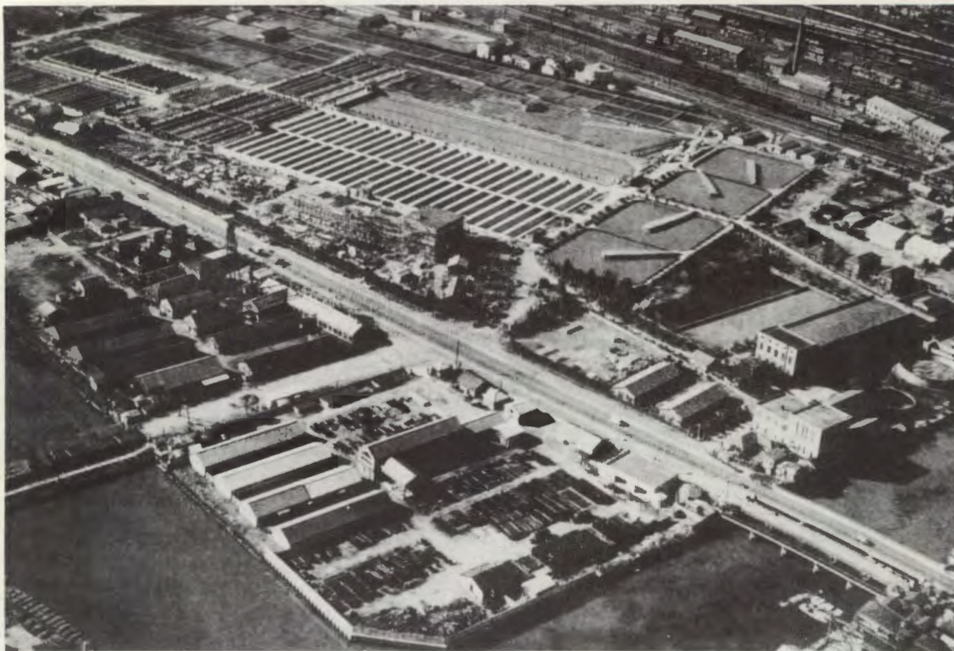
Figure 7-7. Sewage treatment plant in Tokyo.
