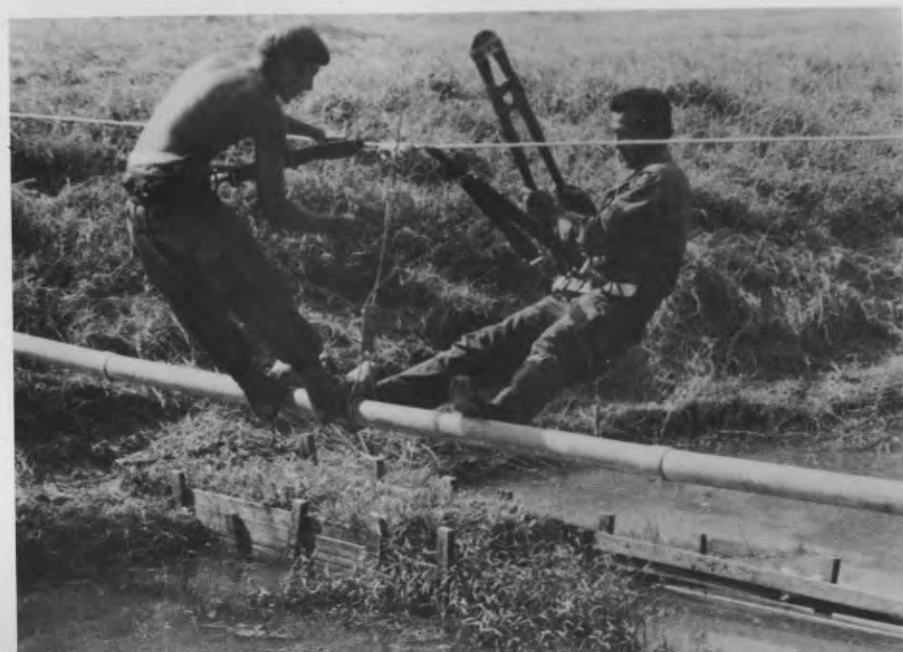
Catenary suspensions provide the support for stringing cable and casings across Thai klongs. Two cablemen from the 40th battalion balance precariously while tightening the bracing cables.
