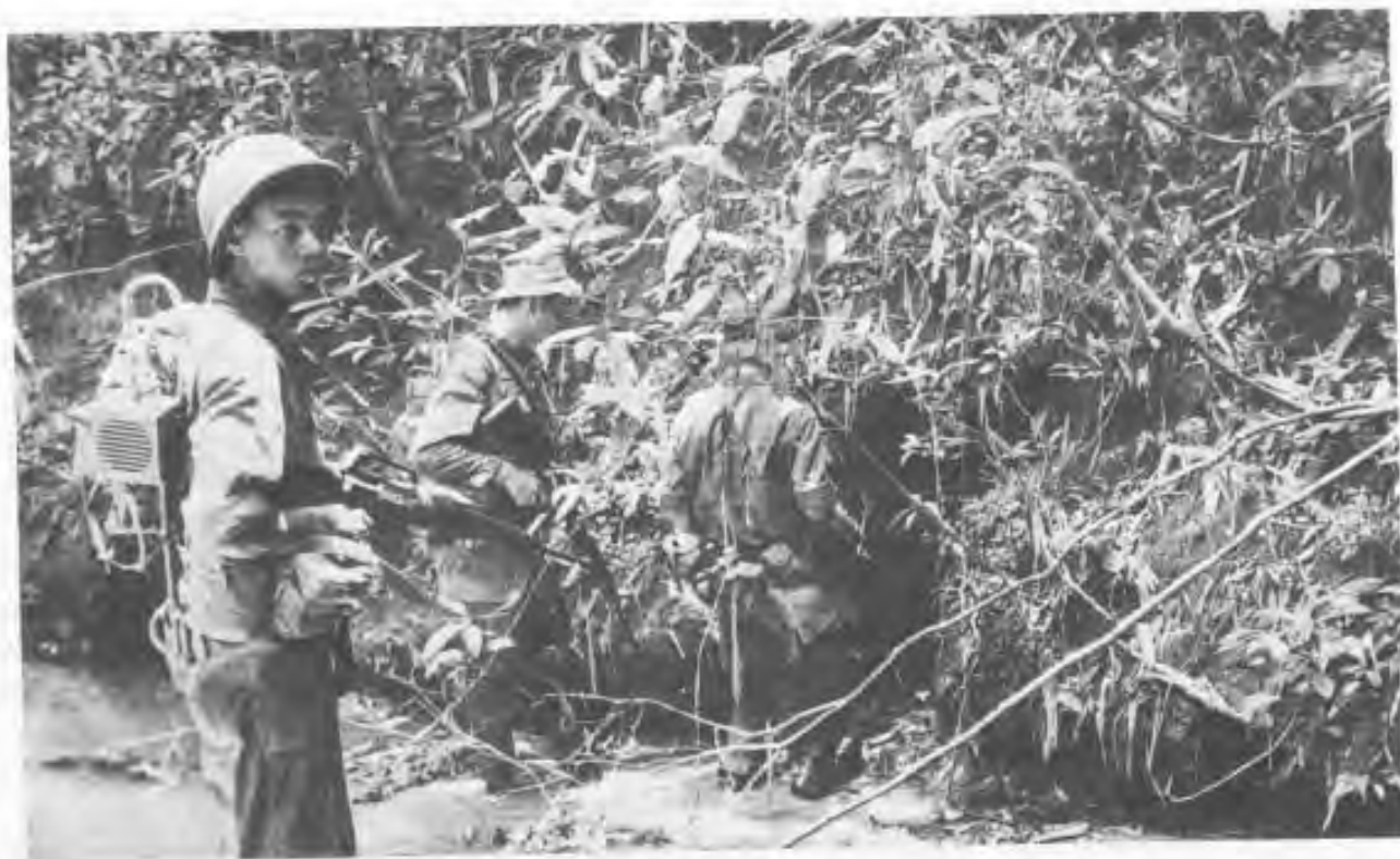
Concealed Tunnel Entrance by River Bank
