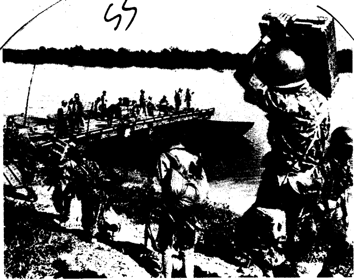
Troops of a joint South Vietnamese-Cambodian task force build a pontoon bridge across a river near Highway 7, about 33 miles southeast of Phnom Penh, where Communists had destroyed a bridge. The bridge materials were flown from Saigon on two U.S. Air Force C130s. (UPI)
