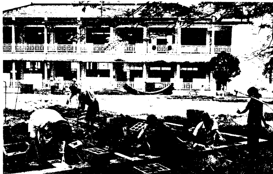
Laborers go to work on a foundation for a prefabricated hospital, one of many such facilities included in the Viet-Nam Ministry of Health's accelerated construction program. AID contributes annually more than $12 million in medical supplies and equipment to support the Vietnamese health program.
