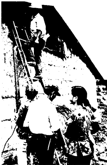
A Vietnamese family watches the installation of electric lines in their home. Membership in one of three pilot rural electrification projects initiated in 1970 costs only 100 piasters (about 25 cents) per family.
