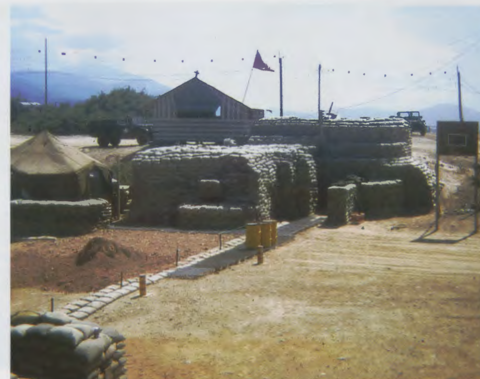
Radar Operations Bunker, Cherry Hill Site – Chu Lai. The back portion, partially buried in the hill, is the operations portion with the radar control unit. The front were two sandbagged Conexes, one for storage and one used for sleeping when rocket or mortar attacks were predicted. We thought the bunker could take a direct 122mm rocket hit. Thankfully it was never tested.
