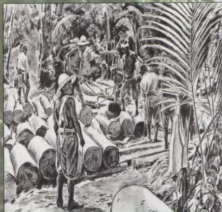
Natives cutting coconut logs for use in fortifications.
