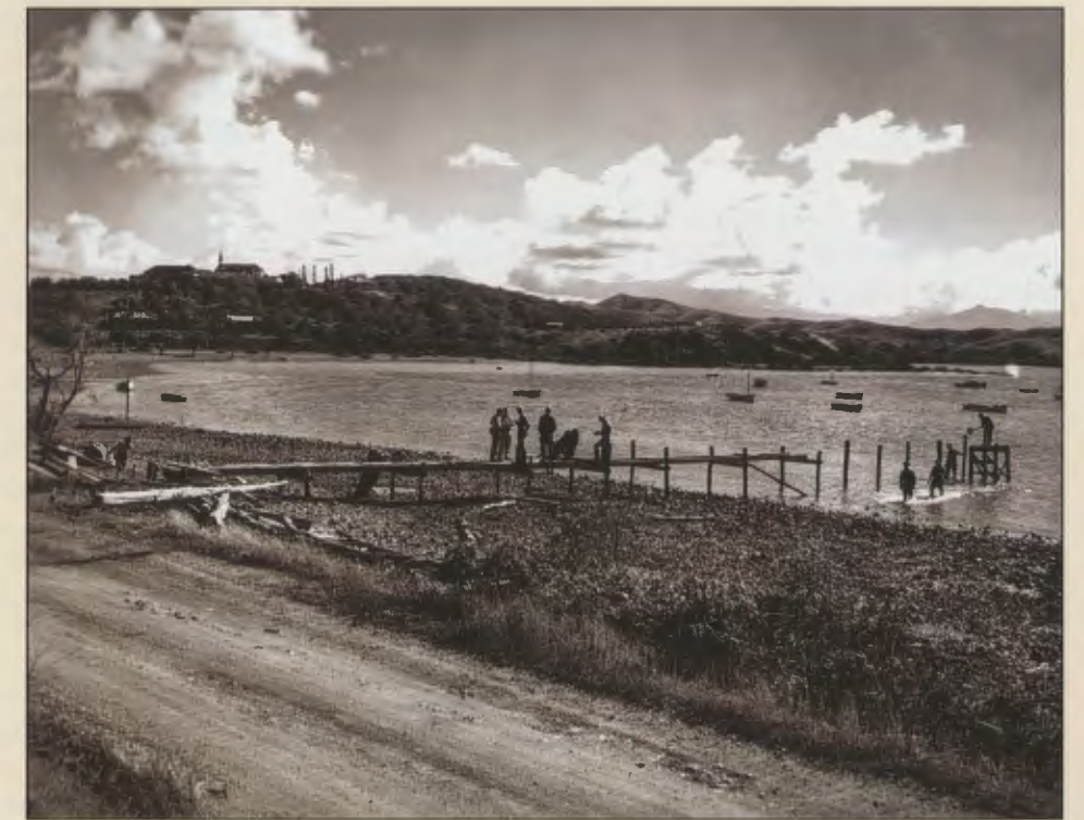
Americal Division, New Caledonia. Task Force 6814 engineer project at Port Des Pointes, Noumea, New Caledonia. Dock being built for loading of gasoline and supplies for the 244th Coastal Artillery Regiment located nearby. 20 June 1942. Photo by U.S. Army Signal Corps.
