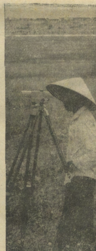
FUTURE RAMP SITE — Water and mud stand in the field soon to become a 100,000-cubic-yard Air Force F-100 Supersabre jet parking apron. Sand is being dredged from nearby Dong Nai River and pumped to the air base to be used as fill. Here, a Vietnamese surveyor checks dimensions for the big ramp. (USAF Photos).
