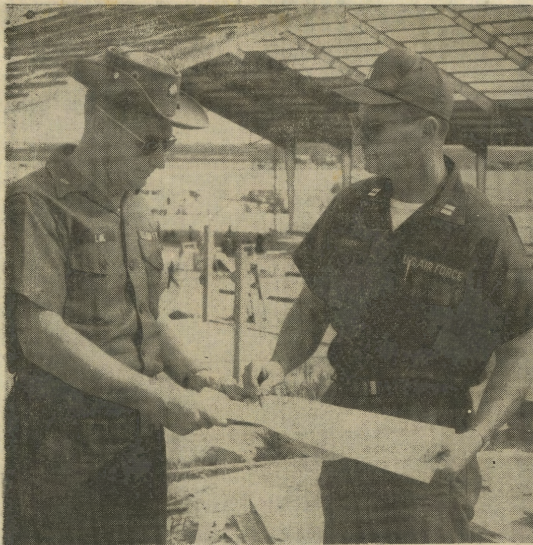
CONSTRUCTION — Air Force Maj. John C. Lane, deputy base civil engineer at Bien Hoa Air Base (left), discusses the new 20,400-square-foot A-1H Skyraider maintenance hangar in the background with Capt. James N. Hicks Jr., construction engineer. The hangar is one of many Air Force facilities under construction at the base.
