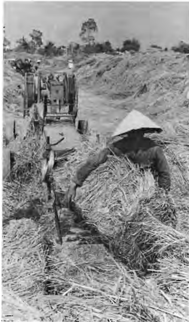
One of the 36 balers under contract to Mr. Nguyen Ngoc Cuong packs straw at its farm location for subsequent shipment by barge to the Cogido Paper Mill in Bien Hoa. Mr. Cuong pays 2,600 piasters ($22) for a ton of the baled straw which otherwise would have been burned by the farmers. A hectare (2.5 acres) can produce four metric tons of straw. The straw is converted into pulp for paper-making.
