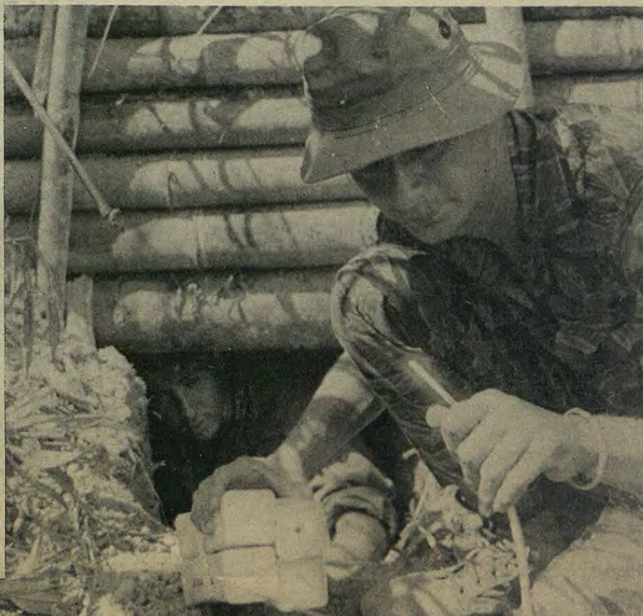
SP4 Dan Jennings, "Demo Man" With The 4th Engineers, Primes A Demolition Block For Destruction Of An NVA Bunker.
