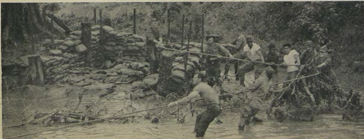
Engineers Strain To Tighten A Cable Over The Dak Psi River As The First Step Toward Building A Bridge.
