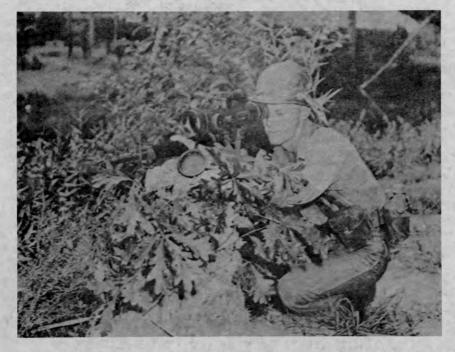
Shown here is the 5-pound individual weapon scope. It permits us at company level to see moving men at over 300 meters under only starlight illumination.
