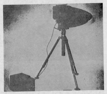
This device, the PPS-14, is a lightweight foliage penetration radar that can give very fine, short range protection to a patrol or an outpost by being able to look through foliage. The PPS-14 is still in R. & D. testing in Vietnam, but looks like a winner.
