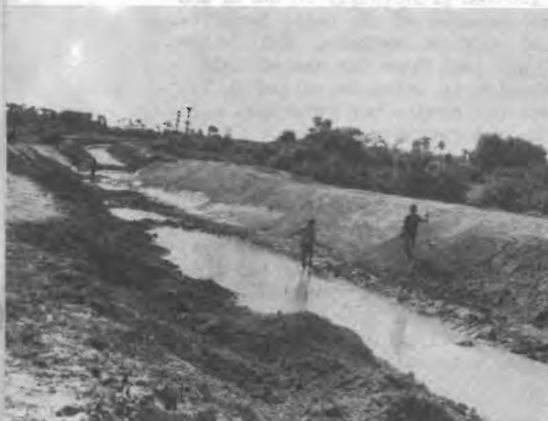
Left : Sodding main irrigation canal to stabilize slopes. Baray, Cambodia. Right : Enlarging main irrigation canal to convey 459 cu. ft. per second. Dragline was furnished by USOM.
