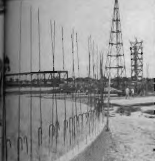
New water treatment and storage plant. Hue Central Vietnam. This new addition consists of a water tower two water tanks and a pumping station which will increased the daily sanitary water supply by 2 642.000 gallons.
