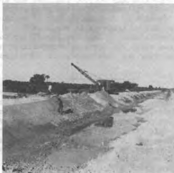
Left : Sodding main irrigation canal to stabilize slopes. Baray, Cambodia. Right : Enlarging main irrigation canal to convey 459 cu. ft. per second. Dragline was furnished by USOM.
