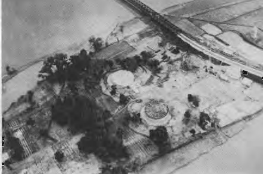
New water treatment and storage plant. Hue Central Vietnam. This new addition consists of a water tower two water tanks and a pumping station which will increased the daily sanitary water supply by 2 642.000 gallons.
