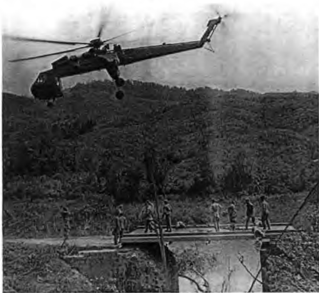
US ARMY PHOTO BY SPS JOHN PETTWAY After delivering a bridge to repair Highway Nine the Cav's Flying Crane moves off for another mission.
