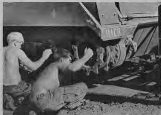
BELLY ARMOR — First Squadron mechanics demonstrate the "book" method of securing protective armor on an ACAV. Innovations in the installation of the 3/4-inch plates which afford added protection against damage from enemy mines, have made it possible to cut installation time in half. (Photo by Cody)
