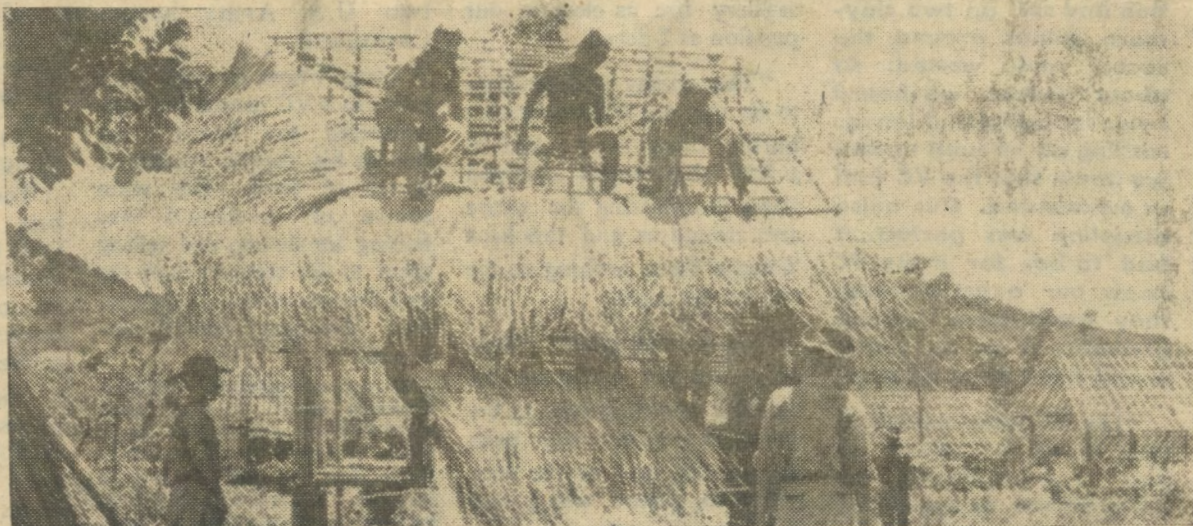
Quy Chanh's construct new home in a government sponsored New Life hamlet.
