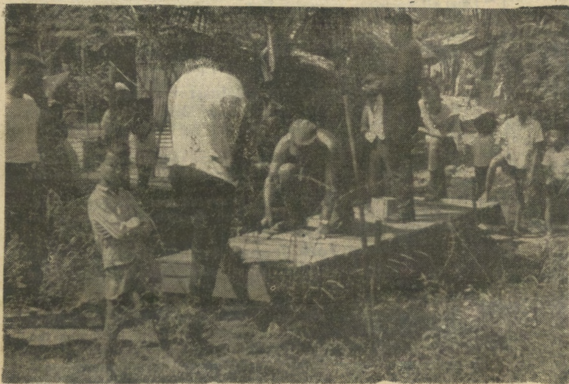
GRAVEL SIDEWALK — What was once a walkway of tires is now an easily negotiated path of gravel, rear, and a single log across a small canal becomes a wide bridge as U.S. advisors on off-duty time nail the final planks on the structure under the watchful eye of several Bac Lieu small fry supervisors. This community project will provide the residents of the city with an easy access to markets, the hospital and center of town.
