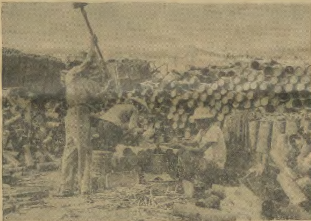
SPIKE JONES — Vietnamese yard worker at Go Vap junkyard uses sledge hammer to drive center pieces out of used shell casings. The two parts are made of different kinds of metal and will be salvaged and sold separately.
