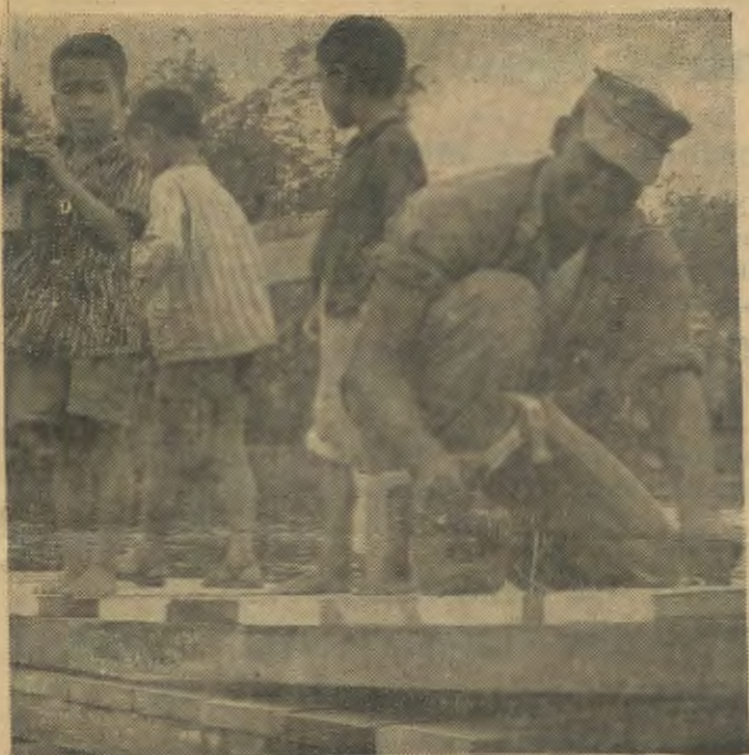
FINISHING THE JOB — Little Vietnamese boys wait impatiently for Marine Cpl. Cornelius A. Smith to finish building a footbridge in the Marble Mountain area, near Da Nang. Marines have constructed many bridges for local villagers. Smith is a member of 3rd Engineer Battalion, 3rd Marine Division. (USMC Photo)
