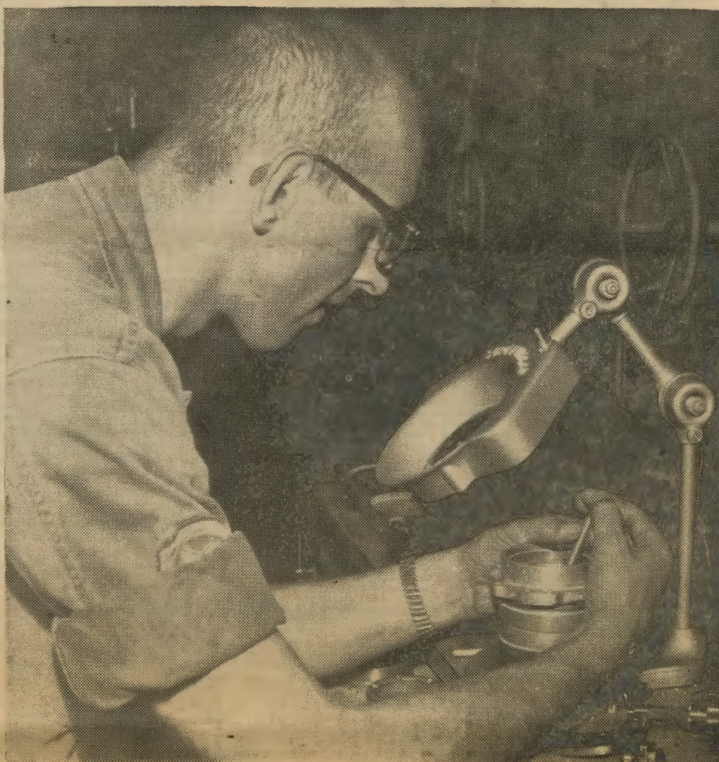
A CLOSE CHECK— A gear box sleeve for a Huey engine, repaired aboard the Corpus Christi, is checked through a magnifying glass to make sure it is ready for installation. Sp5 James R. Sittler removes burrs from the repair job and gives a dimensional check.
