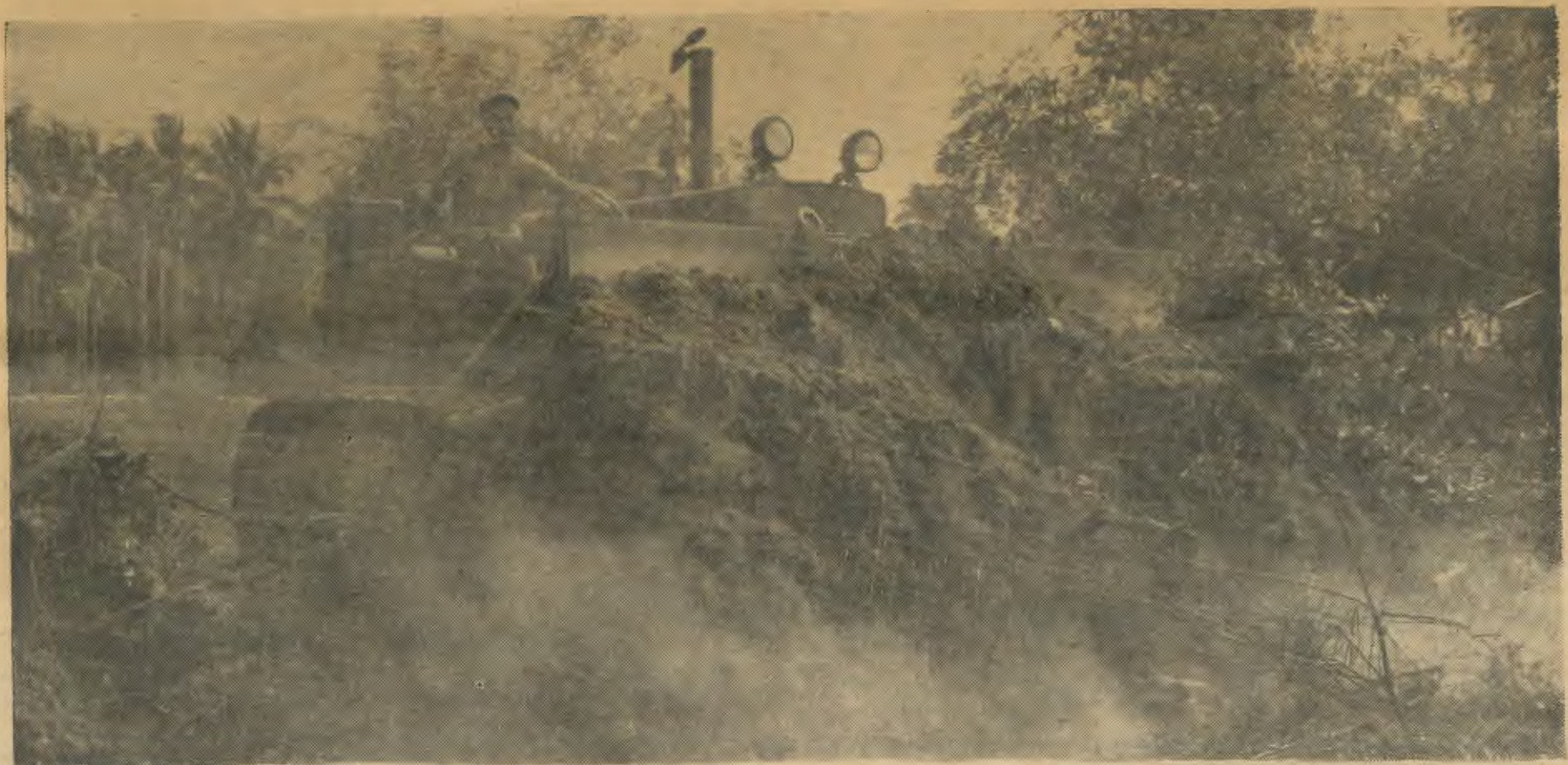
EARTH MOVER — A Seabee equipment operator begins the hard task of turning Vietnamese trails into full size roads. The team has finished one
