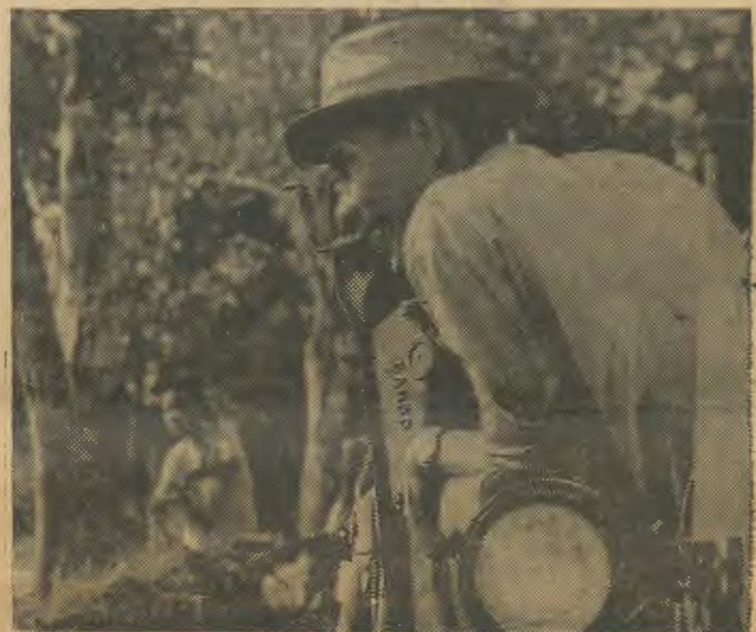
TRAINEES — Vietnamese trainees learn to operate the Seabee's heavy equipment. These are the people that will carry on their own reconstruction long after the team departs.
