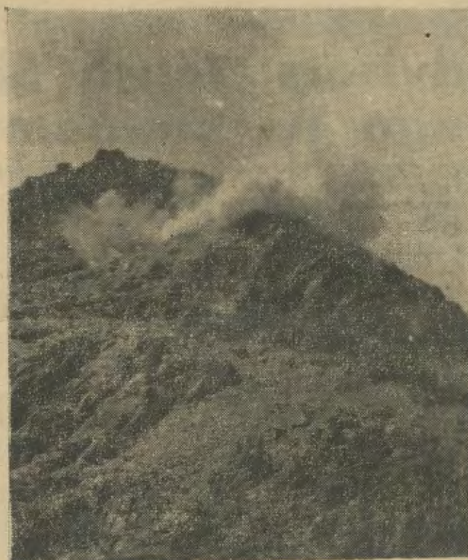
BOOM— A cloud of smoke and dust marks the spot on a mountain where rock for building roads at Cam Ranh Bay is blasted from hard granite. The rock is trucked to a quarry where rock crushers transform it into small rock and gravel for road beds.
