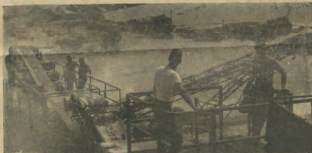
RAISING DUST— Rocks, carried by trucks to a quarry site, are run through this rock crusher where they are transformed into gravel (left) and fine sand (right) by the equipment that raises a constant cloud of dust at the quarry operated by Army engineers.
