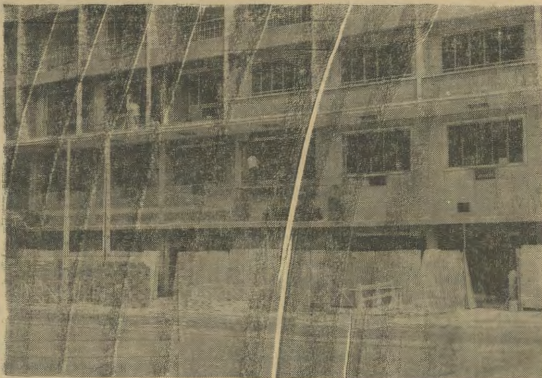
REPAIR WORK PROGRESSES — Repairs to the Victoria Bachelor Officers Quarters are progressing rapidly. Part of the outer walls have been replaced on the three floors which were hit hardest by the explosion that tore through the hotel in the early morning hours of April 1. (See hotel immediately after bombing, Page 4)
