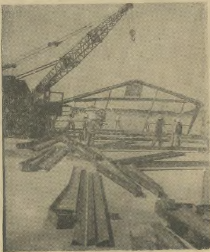
GOING UP — Construction workers from MCB-11 erect 52-ton steel skeleton for one of 15 warehouses at Da Nang East.
