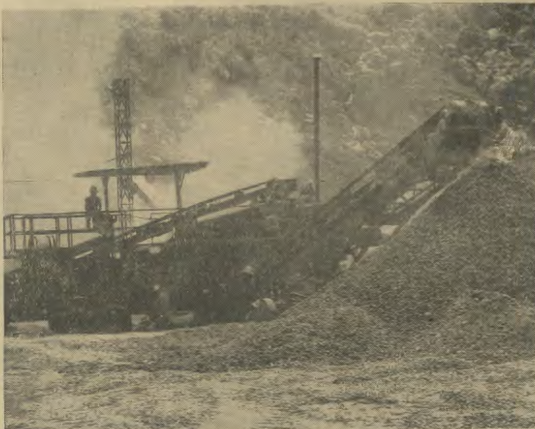
ROCK CRUSHER — Quarrying and operation of this 75-ton an hour crushing plant provide tons of gravel for the battalion's many construction projects.
