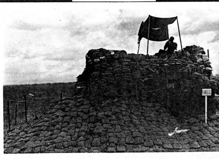
Here's a guy standing day guard with his poncho liner used to protect him from the sun. Bunker #35 is just behind the office. All 8 foot Cyclone Fence is front to protect against grenades thrown by the enemy. There's 3 rows of barbed and concertina wire stretched out in front to protect against infiltration. Note the numerous sandbags and the barrels filled with dirt. Obviously the inside is hollow, and it measure approximately 12 feet by 8 feet inside. Most of them are fairly waterproof, but not all.
