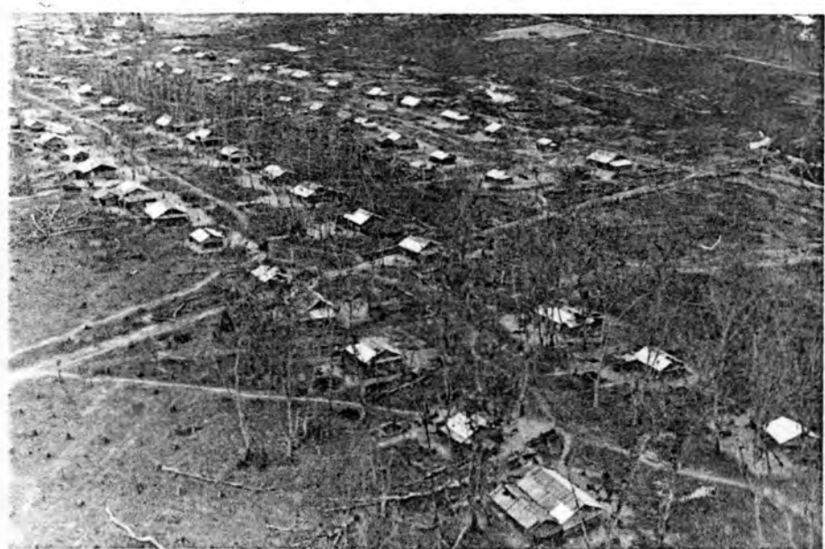
A newly built village just outside Phuoc Vinh. It is unique because the huts are spread apart, and they are normally very close together. Rubber trees are without the leaves (odd, because it was taken in April -- no sign of leafing out). As I recall, I was on a courier mission from Lai Kai to the office that day, and got a pretty wild ride, due to strong winds. We landing at the VIP pad in the middle of the whole complex. That's where the CG's bird lands and takes office, so it's pretty well kept. Note the tin roofs on all the huts, hootches, or houses (your preference).
