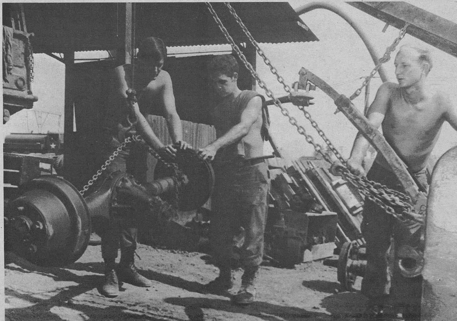
Maintenance replacement includes such large items as a truck differential housing to keep a three-quarter truck operational.
