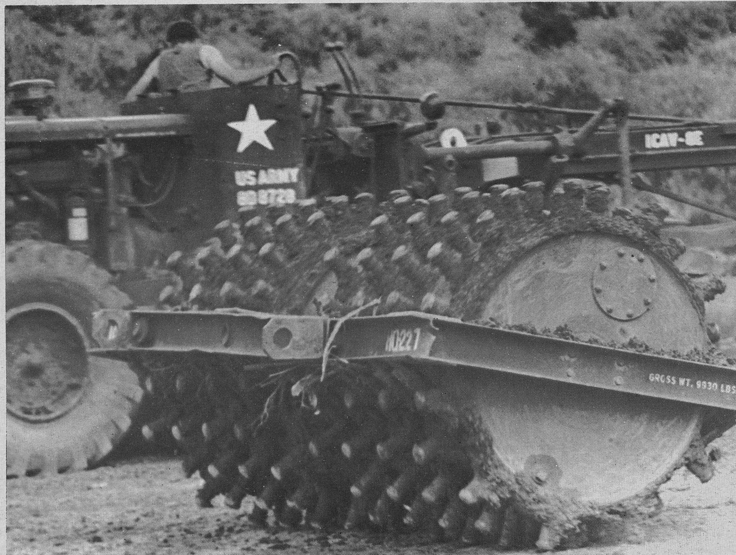
Grading and hardening the soft soil on the runway extension at Bu Dop's air strip is no problem for 8th Engineer personnel with the use of heavy equipment brought into the area for the two month operation.
