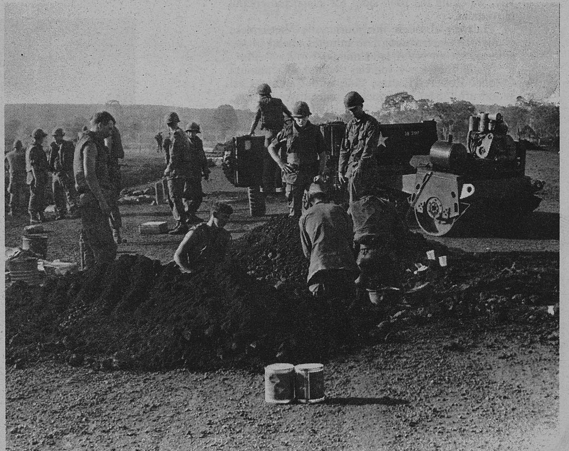
(U.S. Army Photo by SP4 Robert Sharp) Two squads from Company C, 8th Engineer Battalion, patch up the heavily-hit Bu Dop airstrip following a night of intense shelling. The 1st Cav engineers worked around the clock for two days repairing the pock-marked runway.
