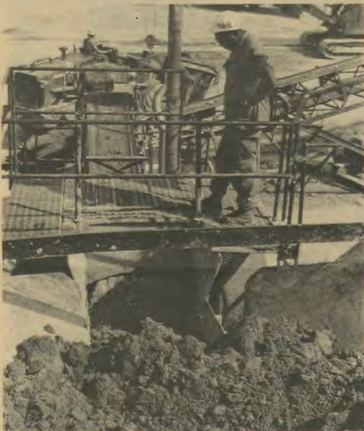
Dirt and rock make their way into the mouth of the crusher.
