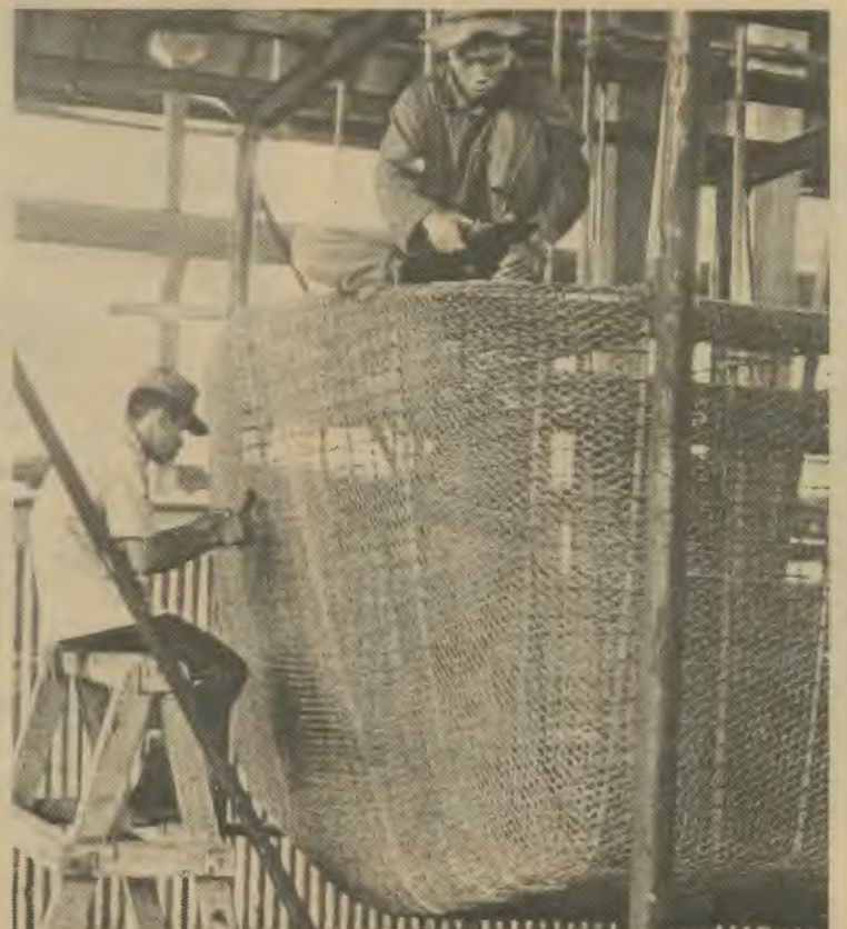
A worker applies finishing touches to the chicken wire and reinforcing rod framework for a ferro-cement craft.
