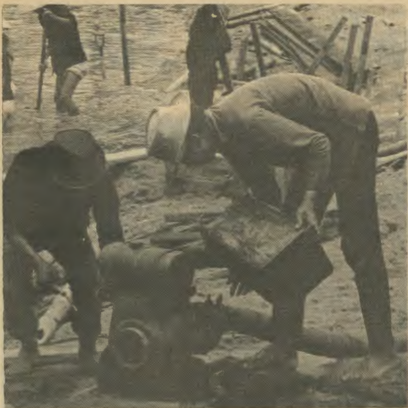
Pumps are employed to expel water from the bottom of the dam, discharging it into the drainage canals.
