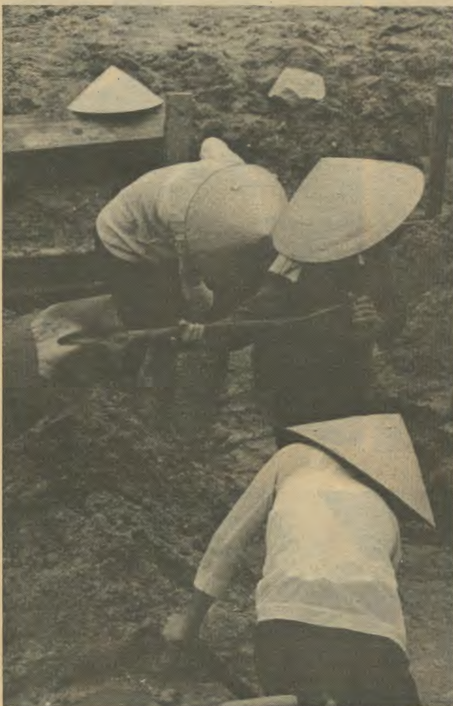
Women laborers scrape mud from the canal to keep water flowing freely, thereby draining the dam site. Drying the construction site makes it possible to build a dam's concrete and fieldstone foundation.
