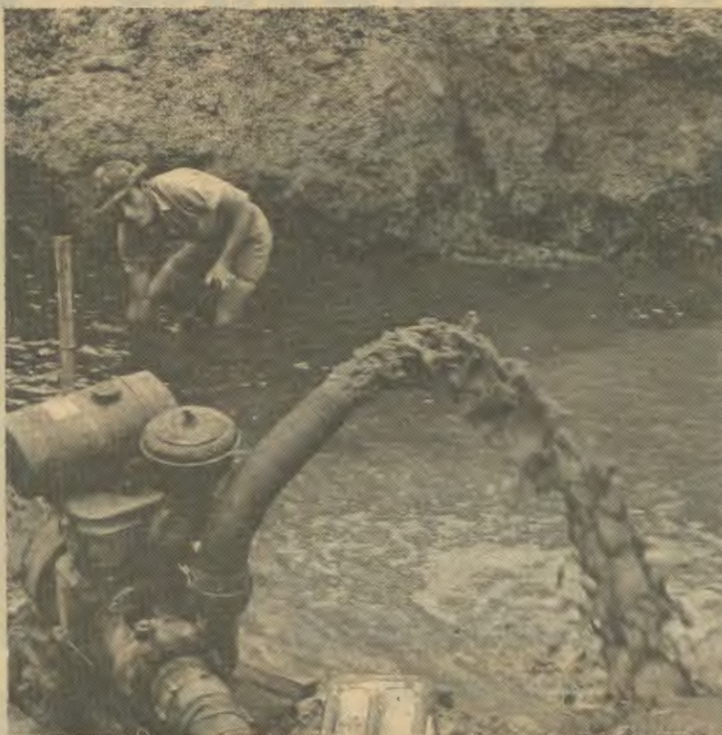
Pumps are employed to expel water from the bottom of the dam, discharging it into the drainage canals.
