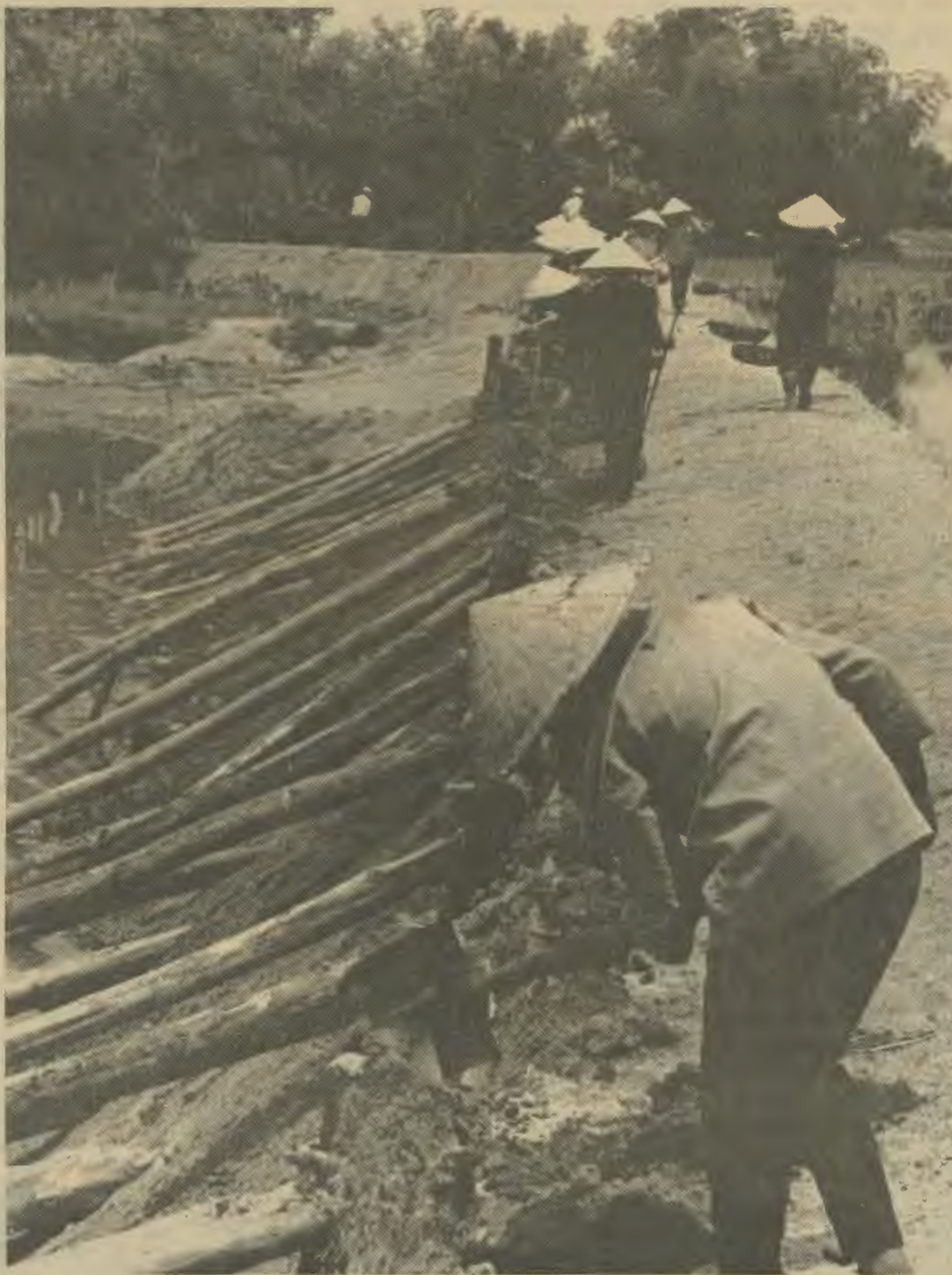
Sand excavated from the sides and bottom of the dam site is deposited behind the reinforced wall.
