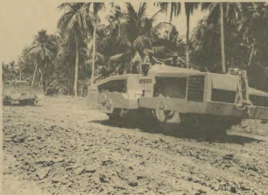
A MAC-LOC compactor prepares the sub-base course of the Cho Gau by-pass.
