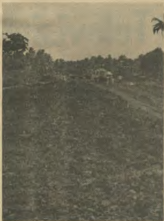
A section of the Cho Gau by-pass shows the extensive use of paddy clay used in the base courses.
