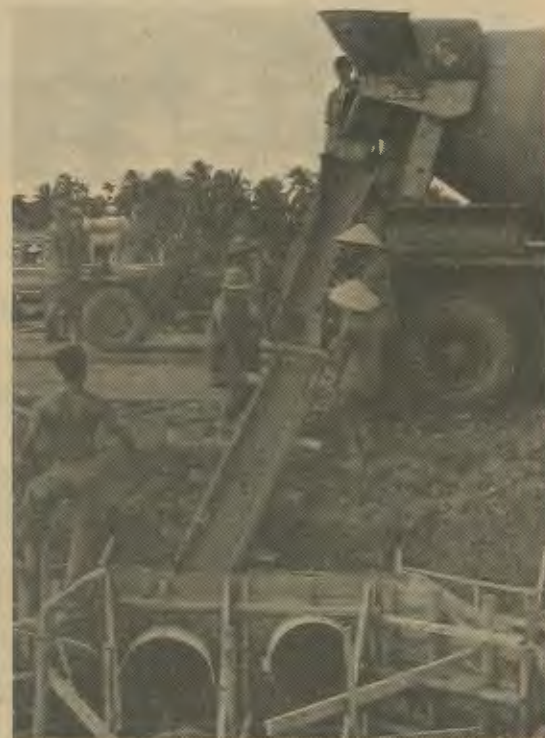
Vietnamese civilian laborers from the 93rd Engr Bn assist in pouring a concrete headwall for one of the numerous culverts built into the Cho Gau by-pass.
