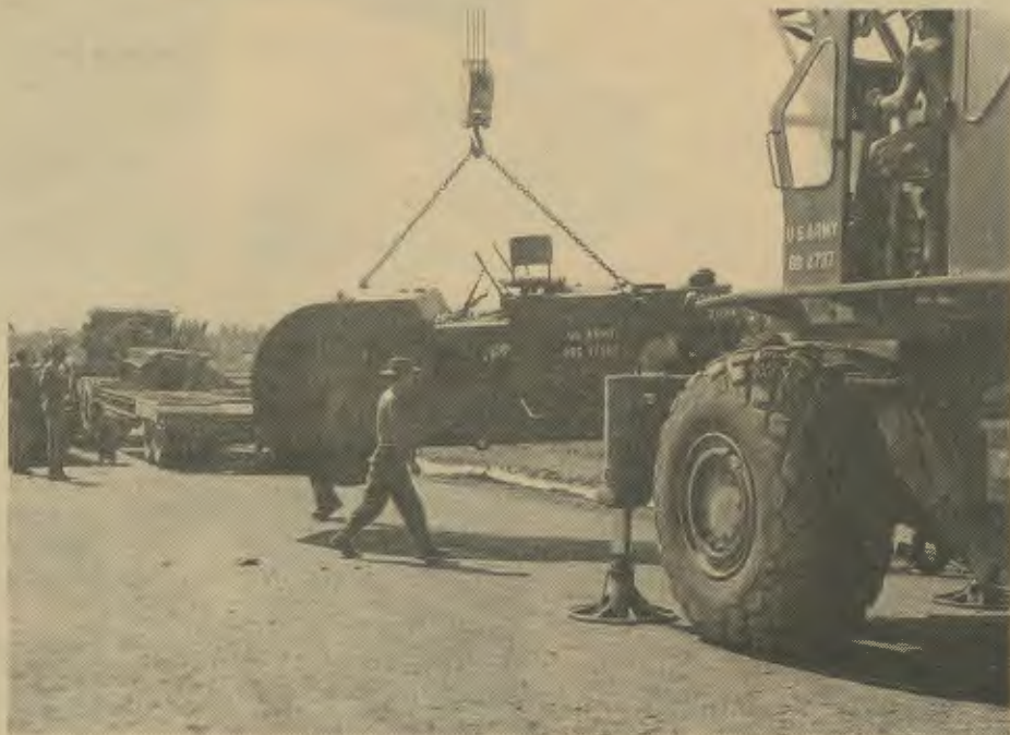
A crane lifts a 10-ton roller during construction of the Cho Gau by-pass.
