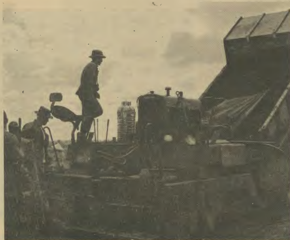
Hot asphalt pours from a truck into a paving machine as the first lift of the Cho Gau by-pass is laid.
