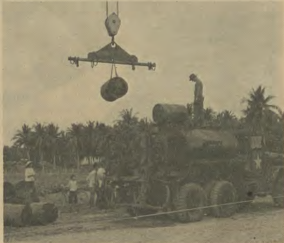
A crane lifts a drum of asphalt paste that will be poured into a penneprime distributor.
