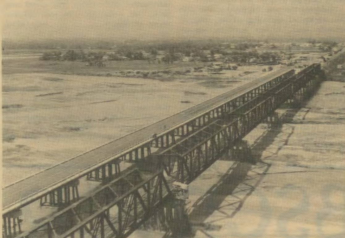
AN INVESTMENT IN THE FUTURE — Bridge QL-1-241 spans out majestically in Tuy Hoa. 3610 feet in length and consisting of 59 spans, the bridge will handle two-way traffic where such traffic has not traveled in twenty years. Built entirely by ARVN Engineers, it was completed forty-five days ahead of schedule.
