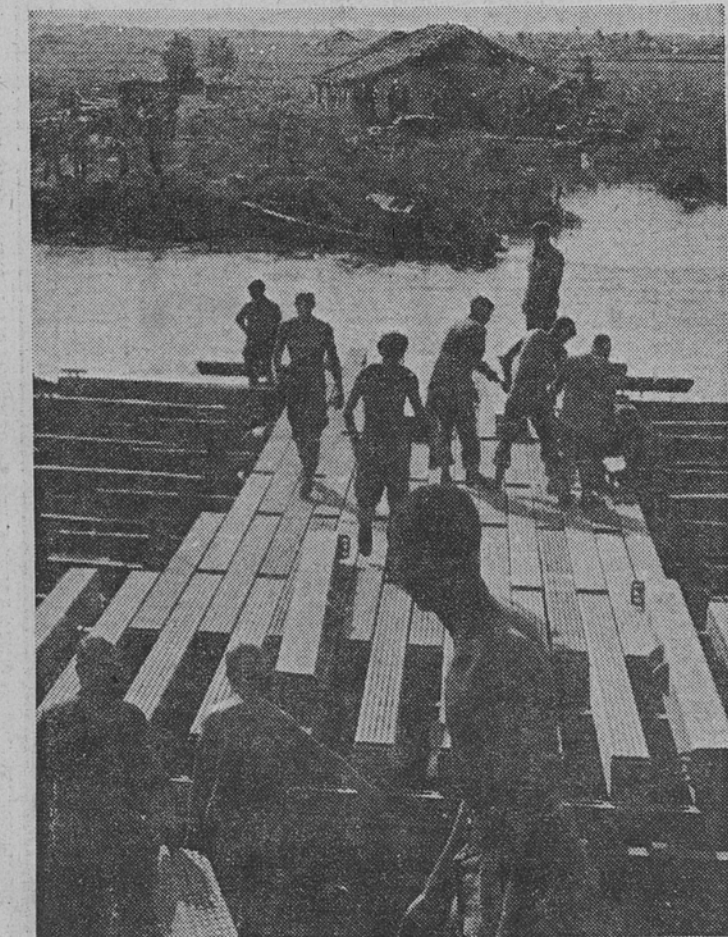
Men of the engineer battalion emplace sections of a bridge.
