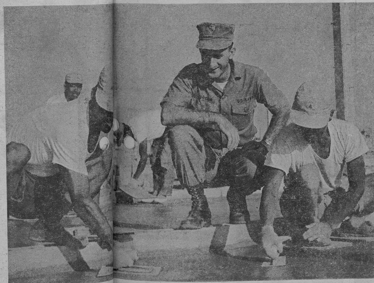
Project officer for the OICC supervises two workers as they finish the concrete floor of one of the units.
