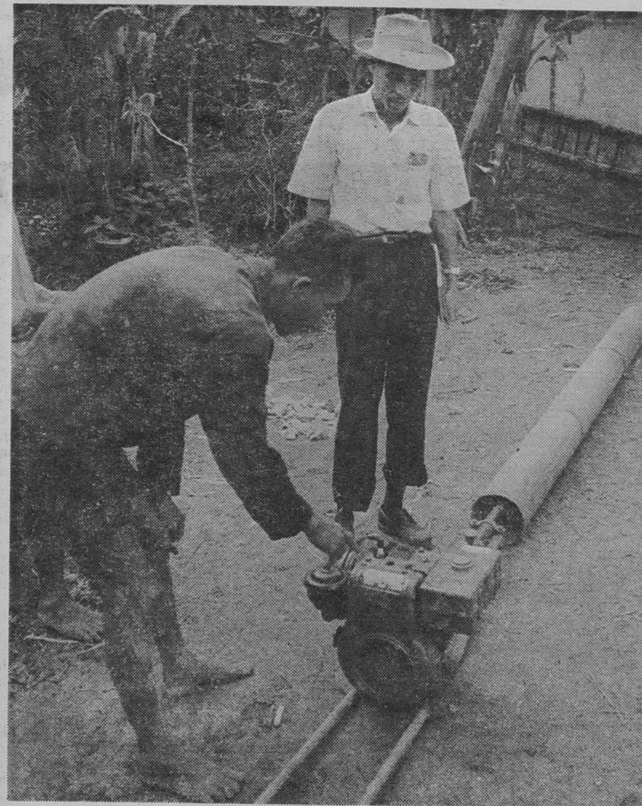
Hoi shows Truong Van Than how he uses an outboard motor as a pump.
