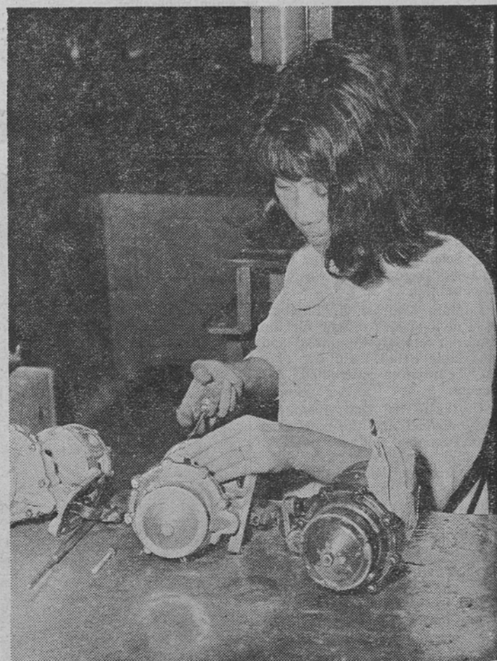
Mrs. Tran Thu Thuy disassembles a fuel pump.
