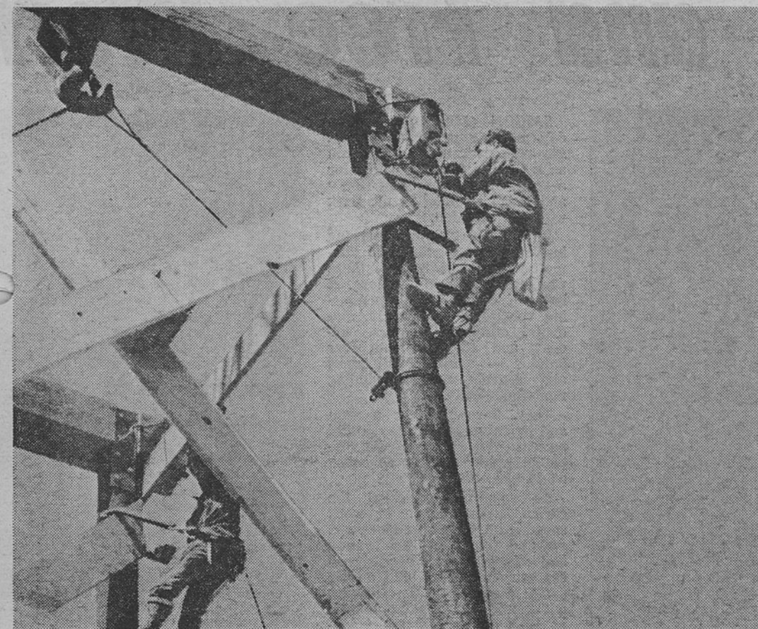
TWO STEEPLE-JACKS HOOK UP CONNECTORS OF THE PRE-FABRICATED TOWER
