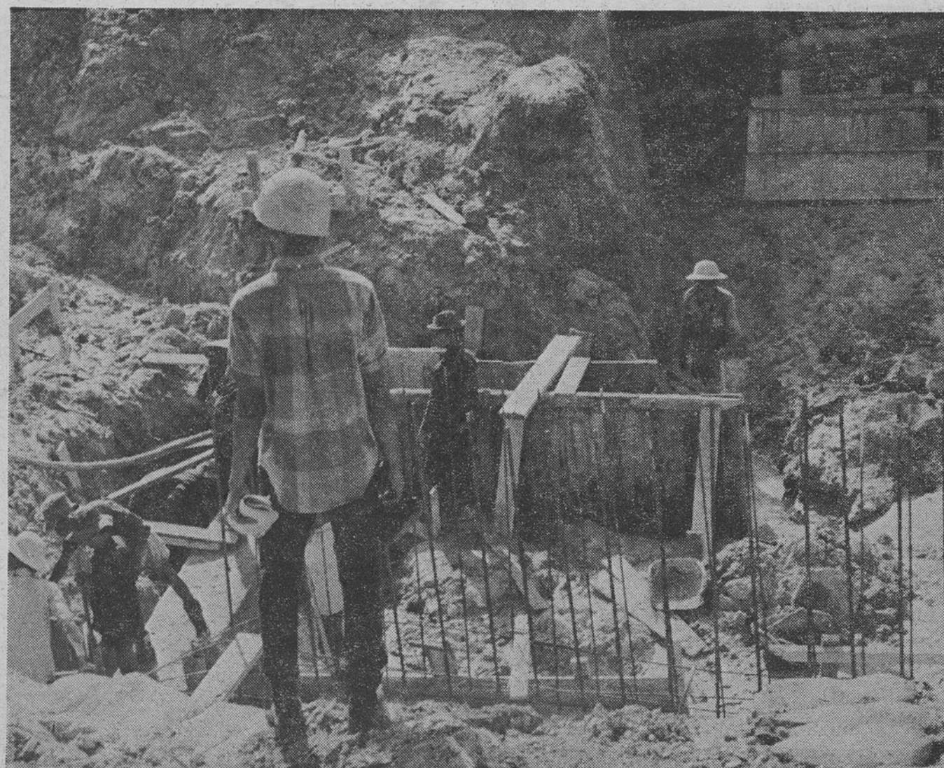
ONE ADVISOR WATCHES AS THE FLOOR OF THE DAM RECEIVES A LAYER OF CONCRETE
