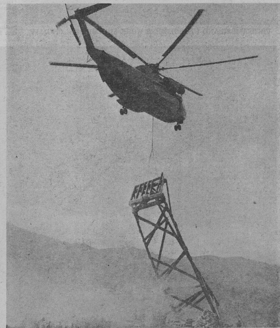
A SEA STALLION HELICOPTER LIFTS A 12,000-POUND TOWER INTO PLACE.
