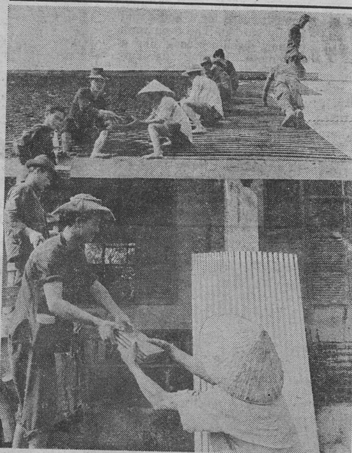
"DISASSEMBLY LINE" —Villagers join together to remove old stone shingles from the leaking roof of Thanh Phu School.
