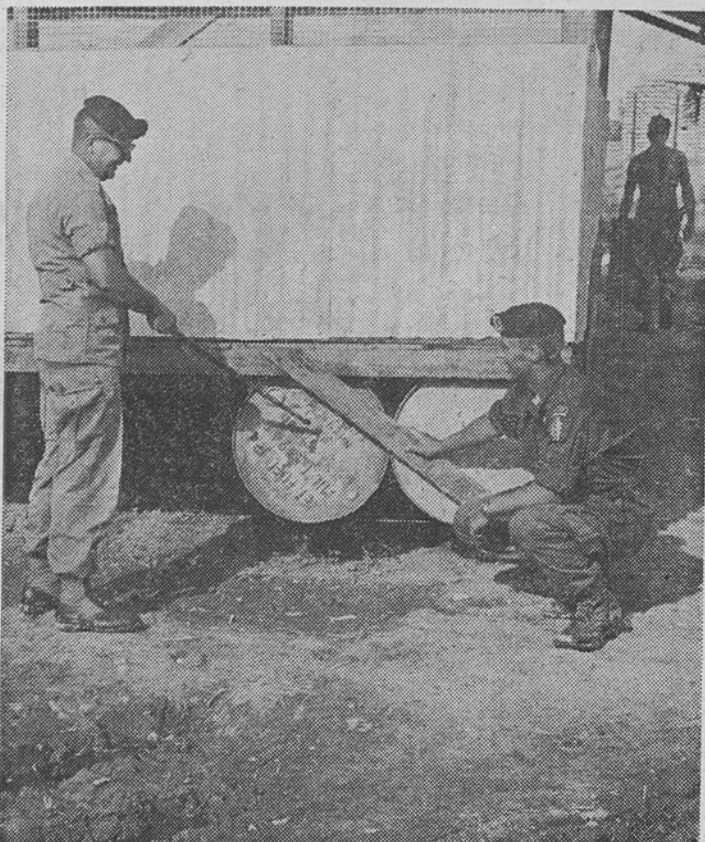
FLOATING BARRACKS —Major J. W. Oliver (left), Collinsville, Ala., points out to Lieutenant R. R. Boaman, Bakersfield, Calif., how the series of 55-gallon drums will float the barracks. (USA Photo)
