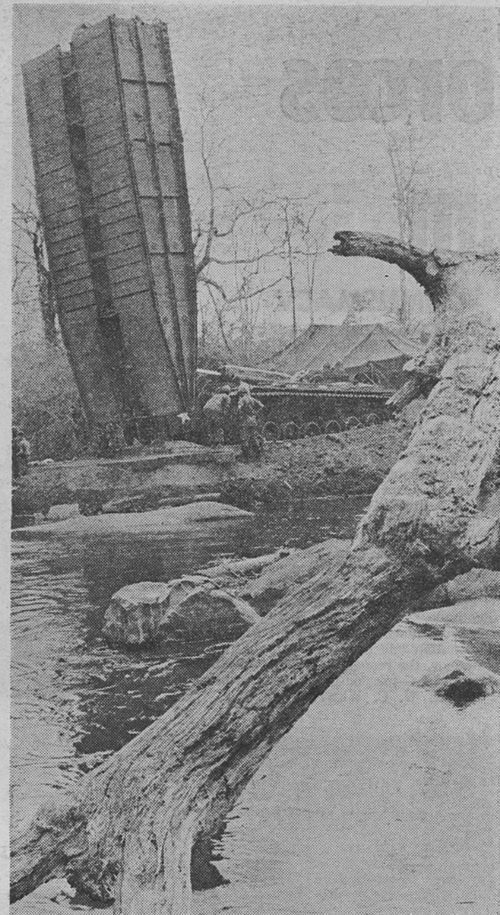
"INSTANT BRIDGES" —An AVLB operated by E Company Engineer Battalion extends itself a 60-foot river,
