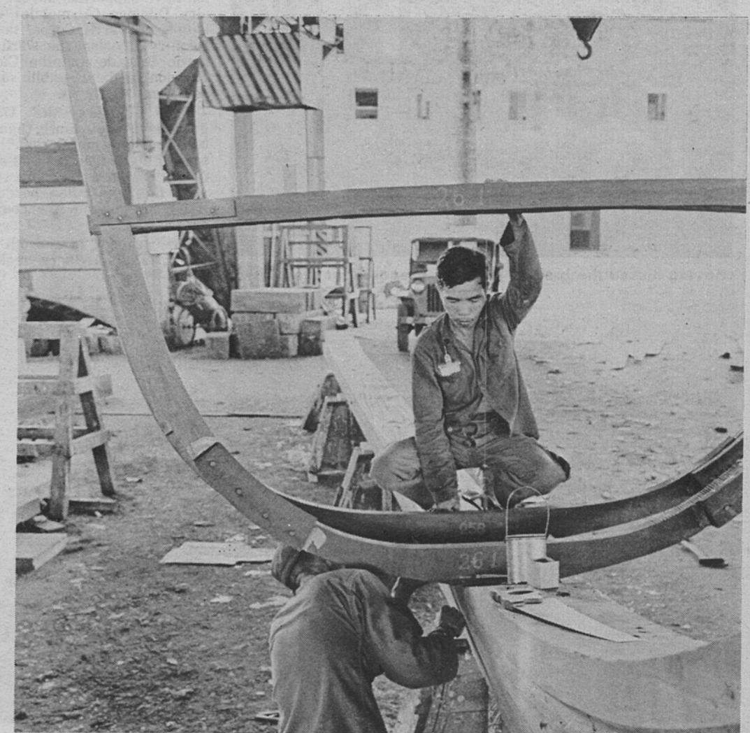
Two Vietnamese boat builders place the first ribs of a junk into place along the keel.
